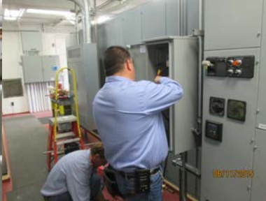
Installation of controls wiring at CCT area.
