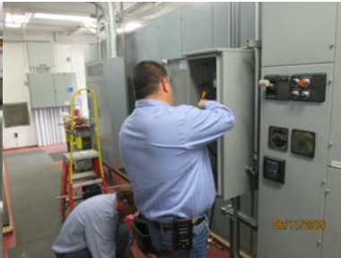
Installation of controls wiring at CCT area.
