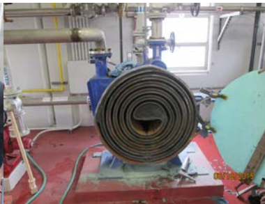
Cleaning the digester sludge heat exchanger
