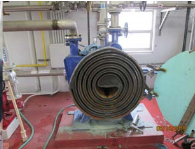
Cleaning the digester sludge heat exchanger
