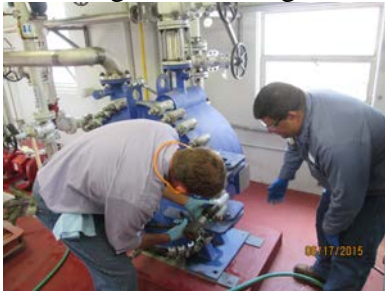
Cleaning the digester sludge heat exchanger
