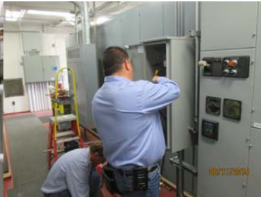
Installation of controls wiring at CCT area.
