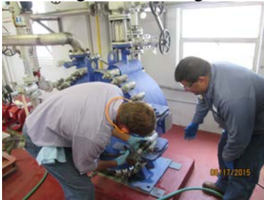
Cleaning the digester sludge heat exchanger
