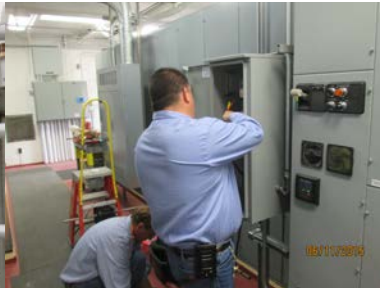
Installation of controls wiring at CCT area.
