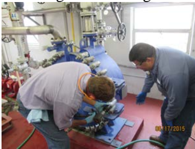
Cleaning the digester sludge heat exchanger
