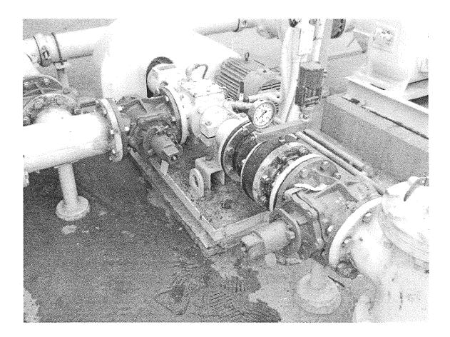
The water filter that will clean the water before it goes to the mechanical seals. This unit will filter down to 50 microns and automatically clean it's self.
