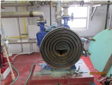
Cleaning the digester sludge heat exchanger
