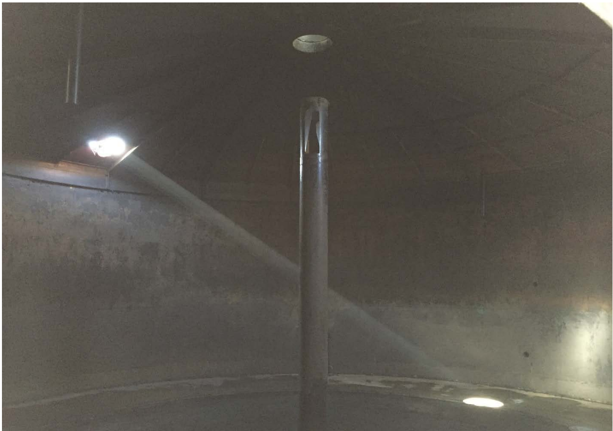
Inside of empty Primary Digester
