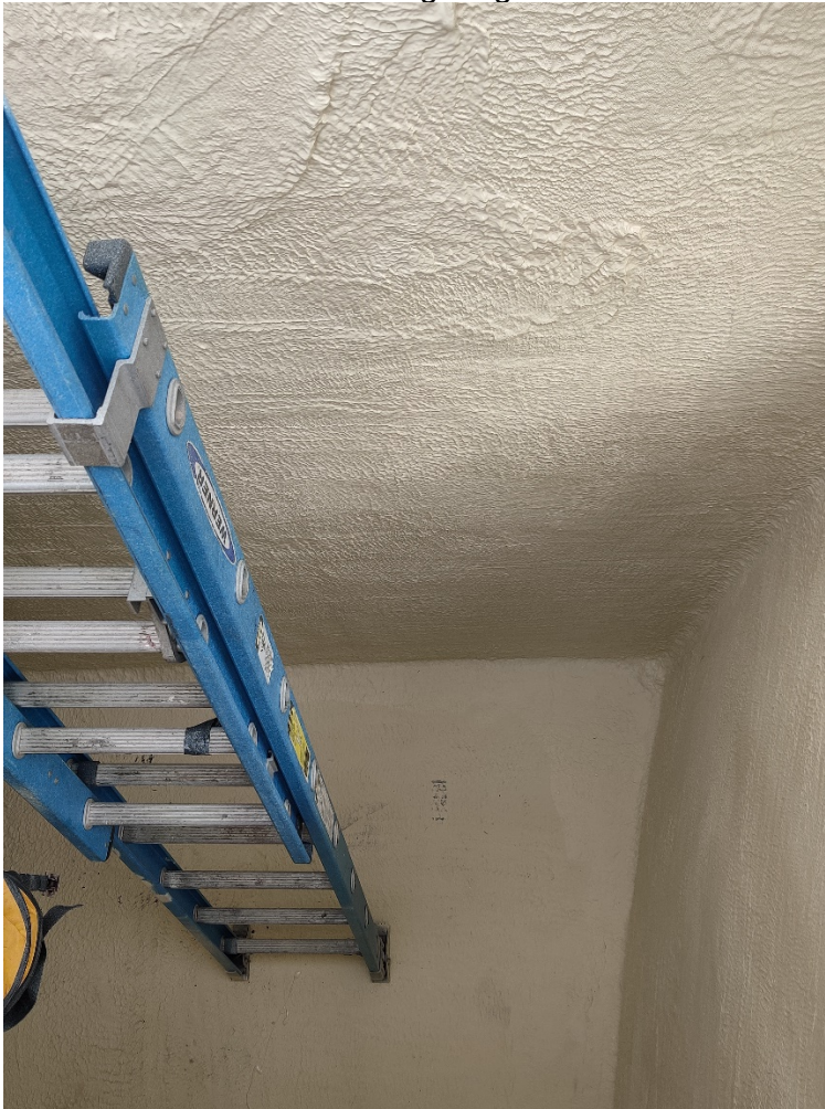
Clarifier launder with rough coating and buildup:
