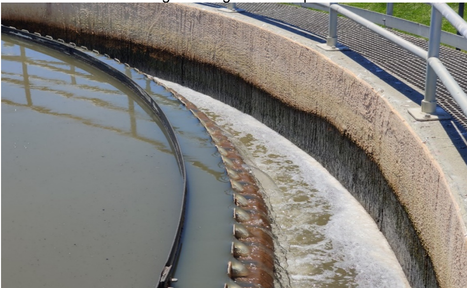
Clarifier launder with rough coating and buildup:
