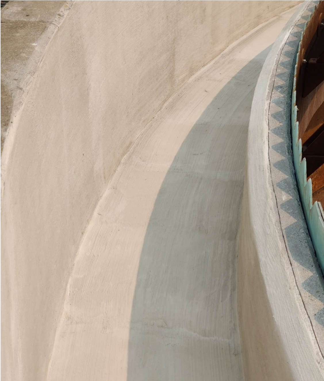
Clarifier Launder Concrete Surface After Resurfacing
