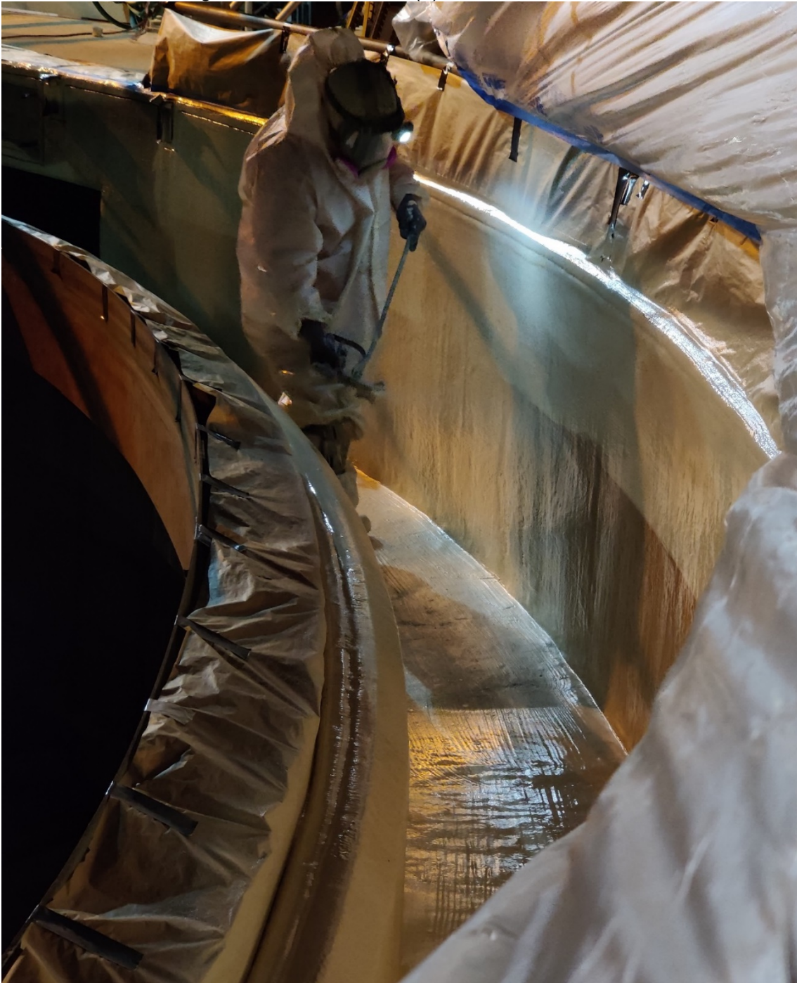
New Clarifier No. 2 Coating with Smooth Surface (2)
