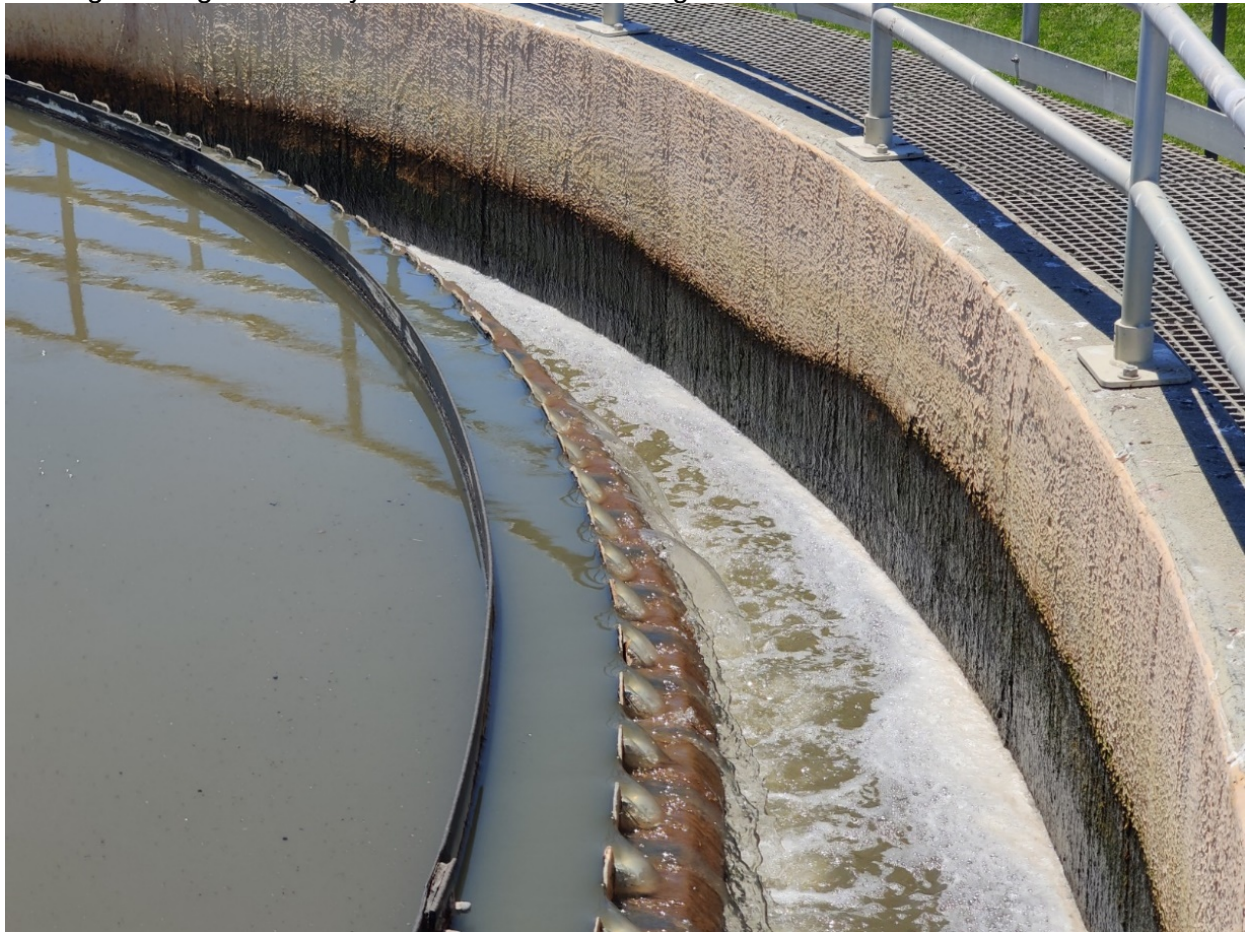
Existing Coating on Primary Clarifier No. 1 with Rough Surface
