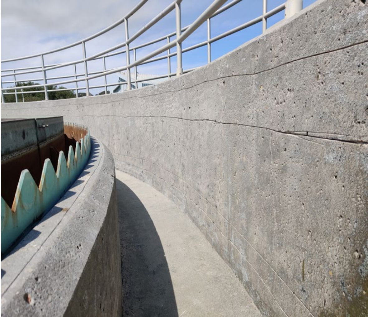
Original Clarifier Launder Concrete Surface
