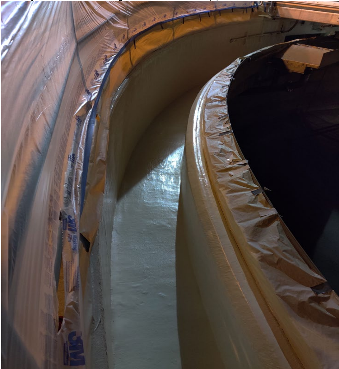
New Primary Clarifier No. 2 Coating with Smooth Surface (1)
