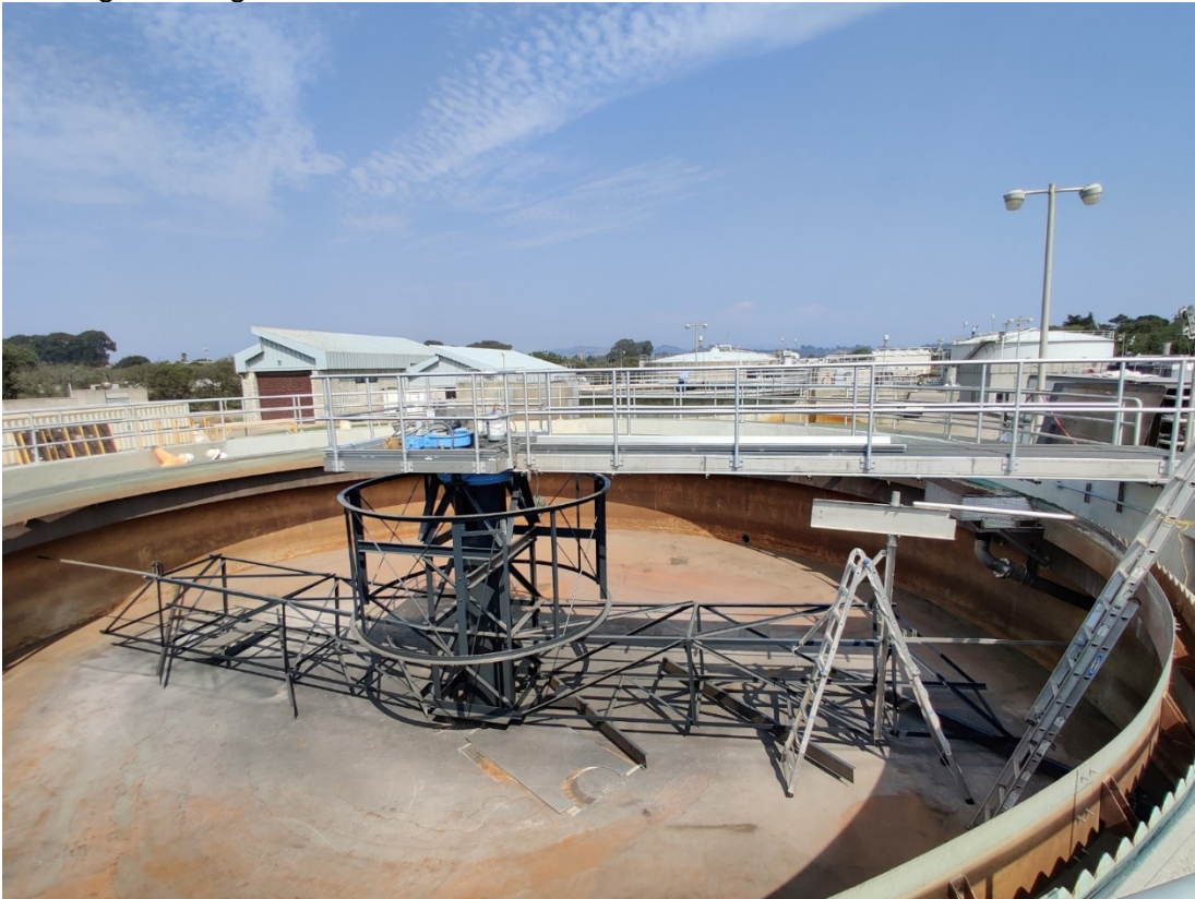
Clarifier Bridge Grating, Aluminum Rails, Kick Plate, and Partial Skimmer installed
