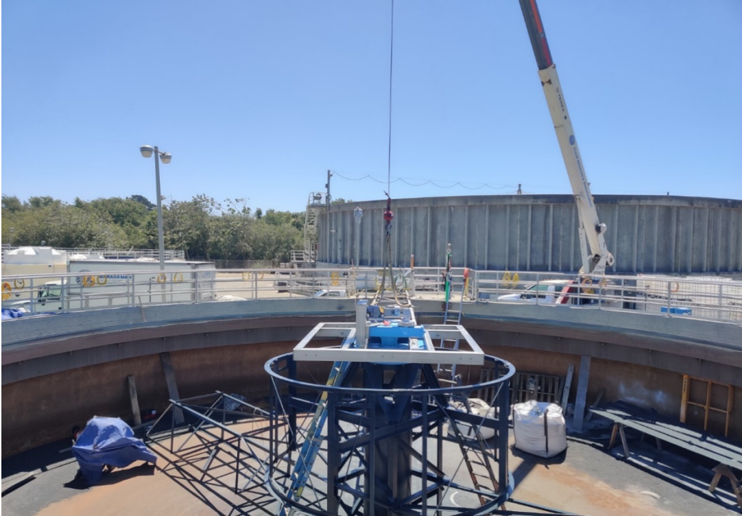
Clarifier Bridge Grating, Aluminum Rails, Kick Plate, and Partial Skimmer installed
