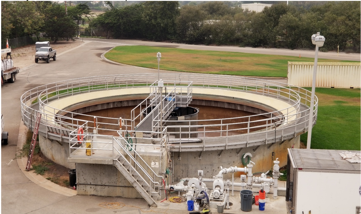
Primary Clarifier No. 2 Near Completion
