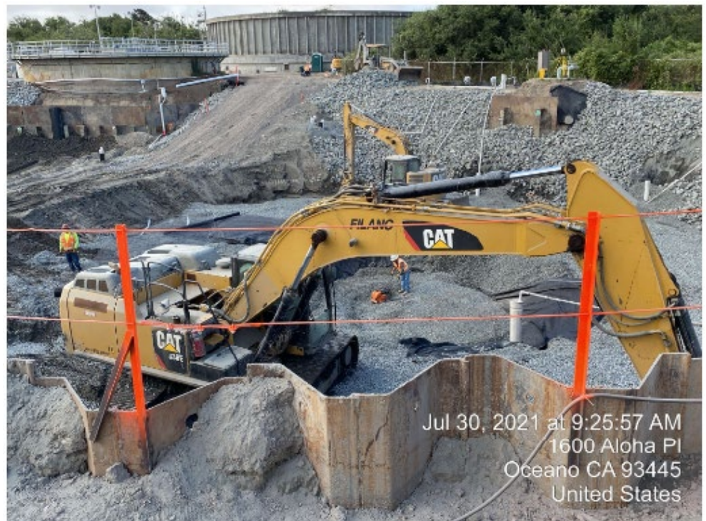
Secondary Clarifier No. 2 Load Transfer Platform Construction_2021.07.30
