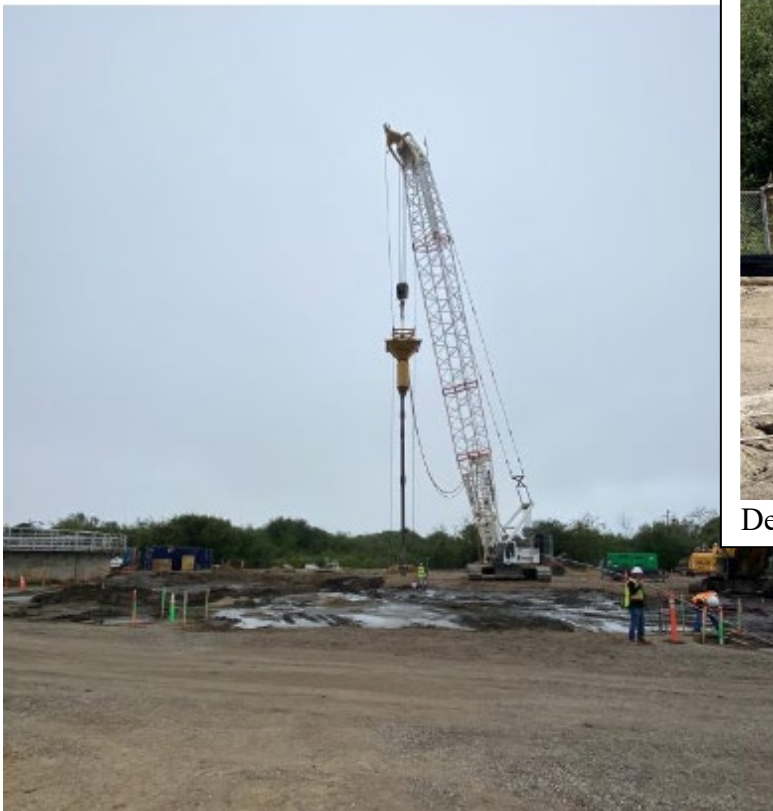
Settlement Monitoring Survey. Vibro-Stone Column (VSC) Crane in background_2021.05.11
