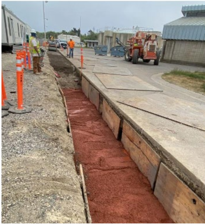
Concrete Duct_2021.05.05
