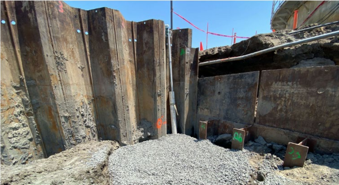
Dewatering Sump Adjacent to Primary Clarifier No.2_2021.07.15
