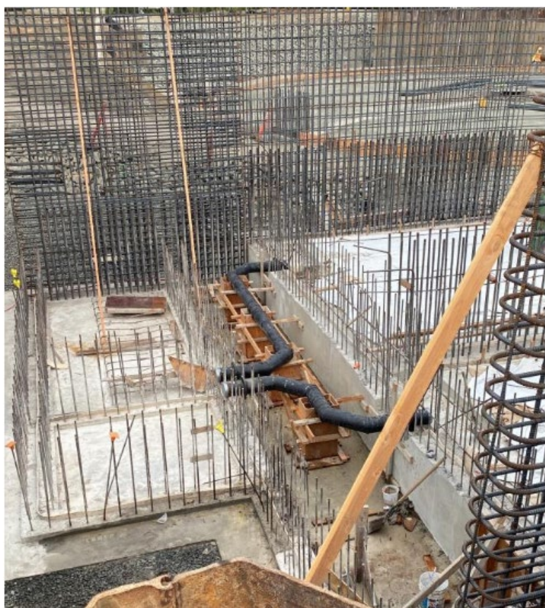
Aeration Basin Drain Piping Pedestal Forms _2021.10.04
