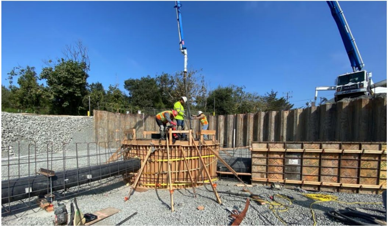
SC2 Center Footing Concrete Placement_2021.08.26
