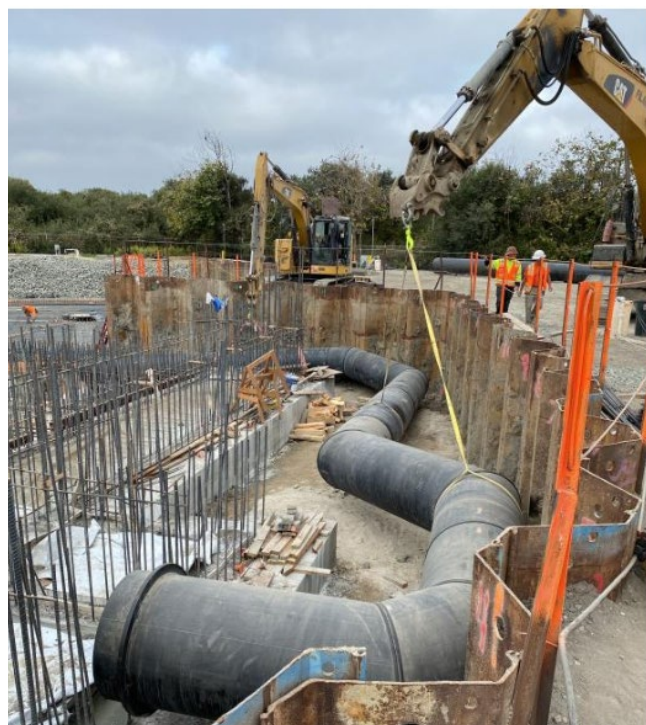
North Aeration Basin 36-inch Mixed Liquor Pipeline _2021.10.07
