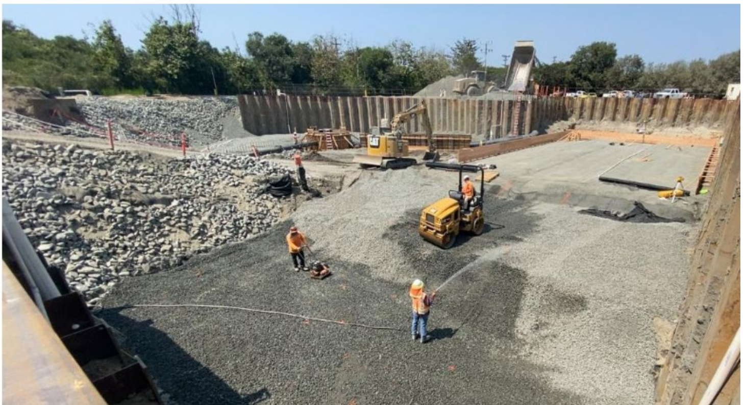
Aeration Basin Load Transfer Pad Installation_2021.08.23
