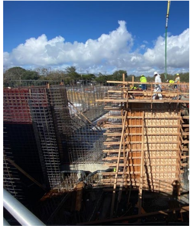
Aeration Basin Concrete Wall Placement 2021.10.25
