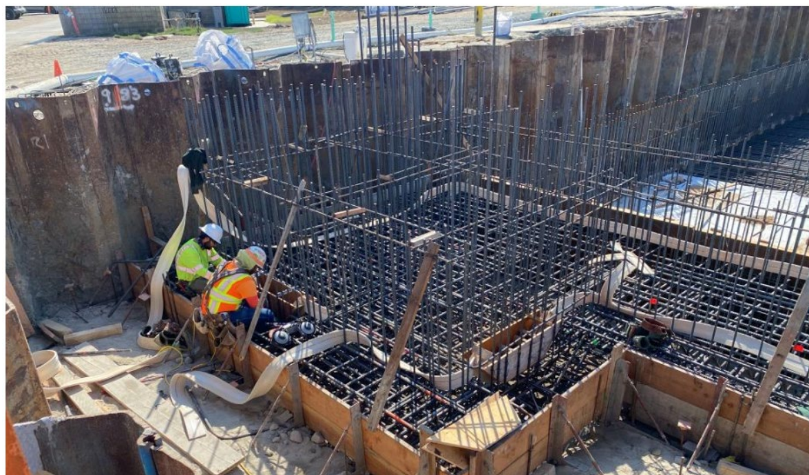
Waterstop Installation at North Aeration Basin_2021.10.01
