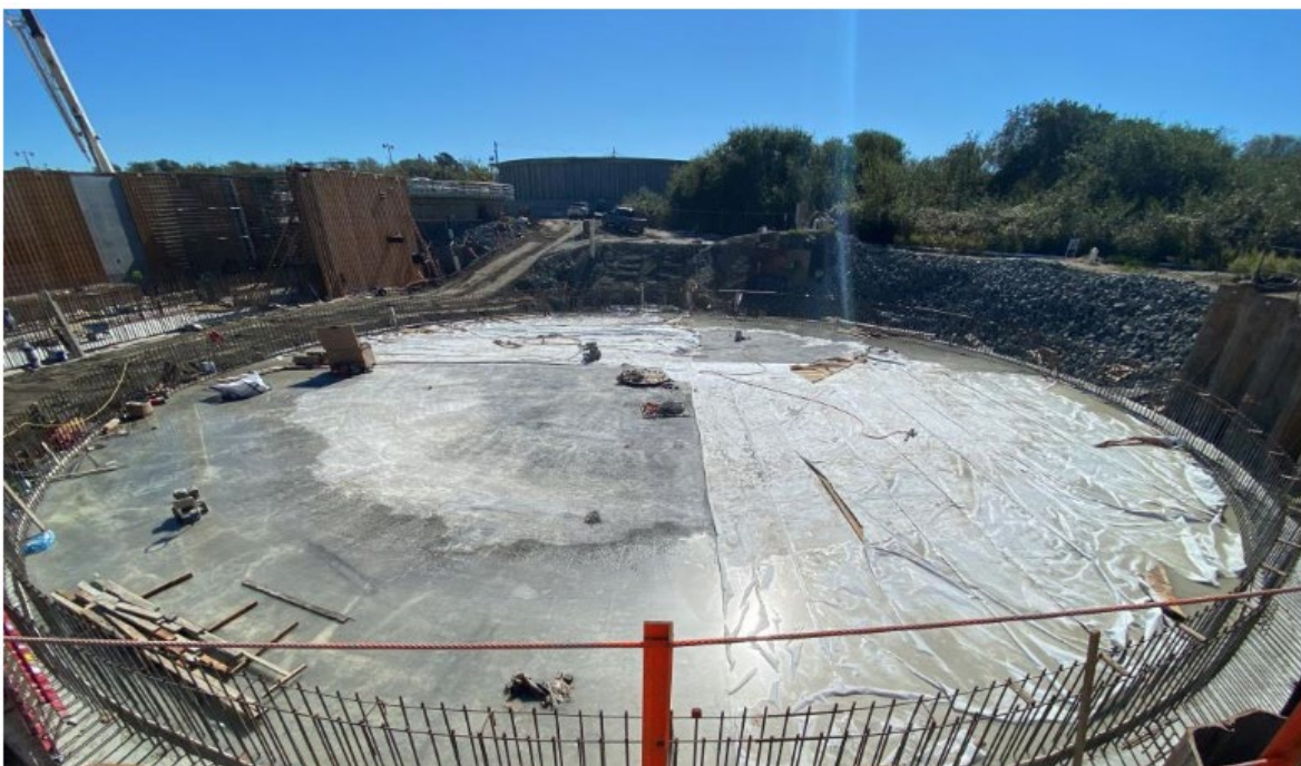
Secondary Clarifier No. 2 Slab Wet Curing_2021.10.28
