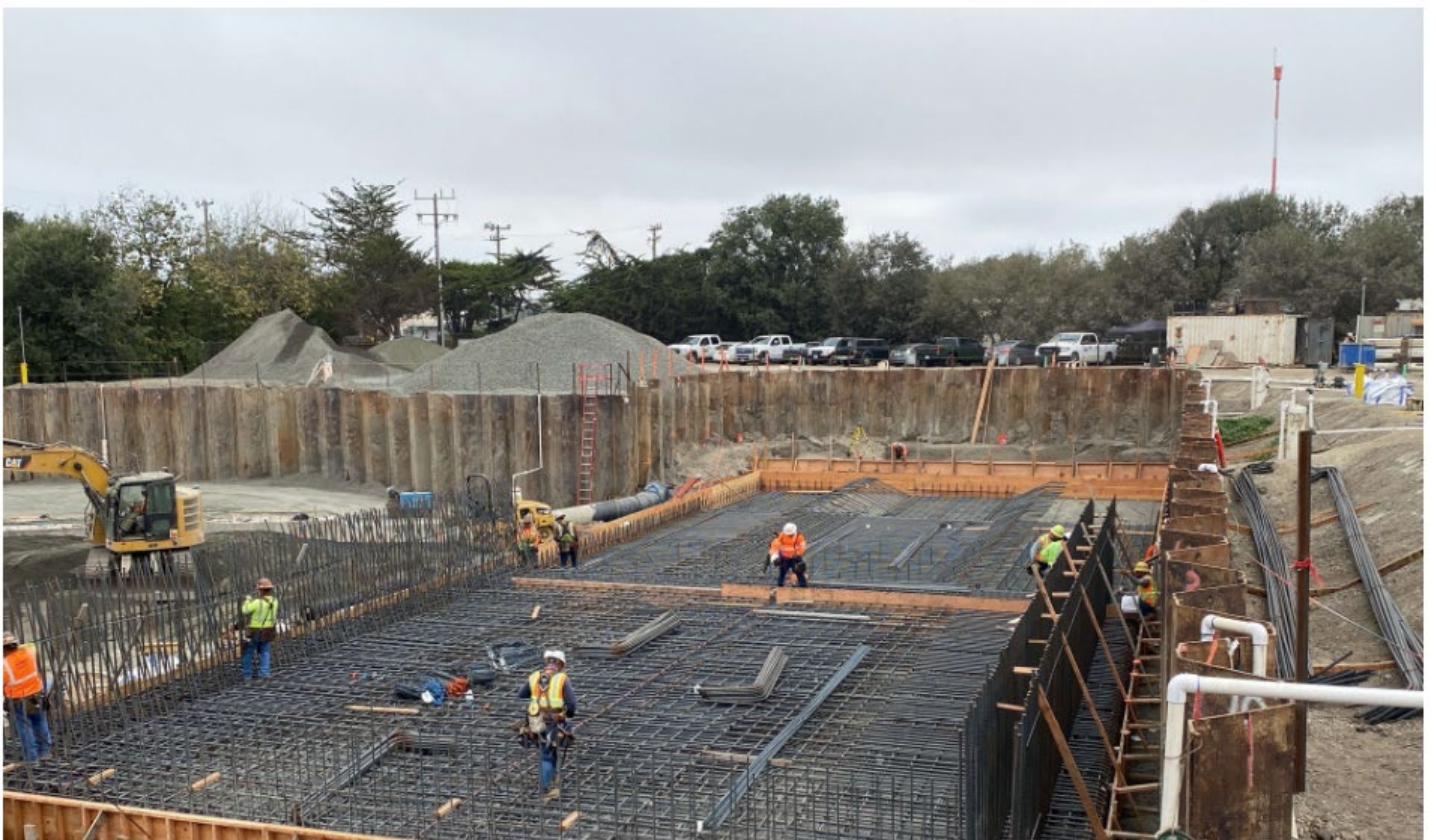
Aeration Basin Rebar Installation 2021.09.10
