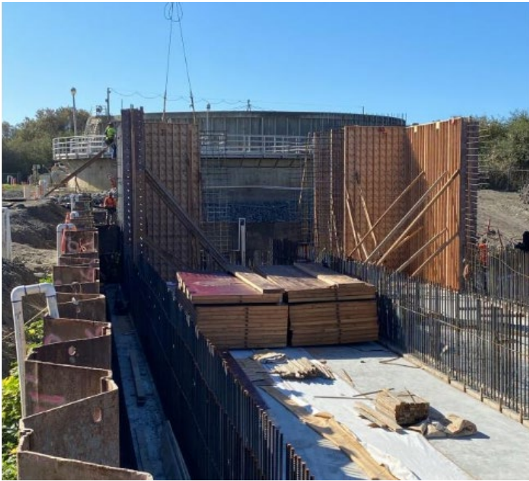
South Aeration Basin Rebar and Forms 2021.10.19
