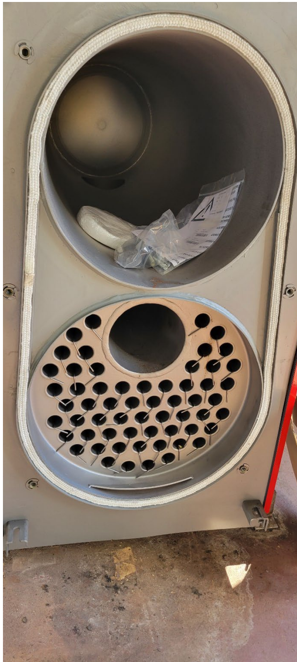
Newly Installed Internal Pressurized Heat Exchanger
