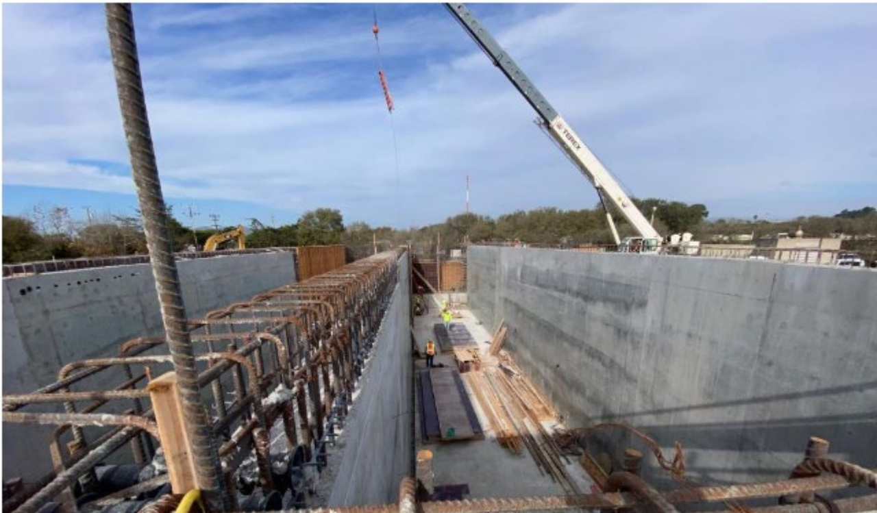
North Aeration Basin Wall Formwork_2021.12.07
