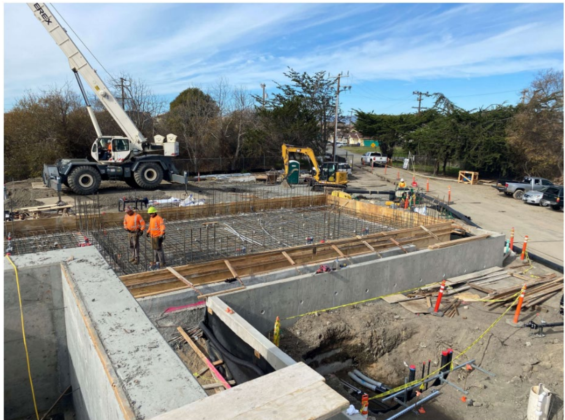
Blower Building House-Keeping Pad Rebar Installation_2022.01.12
