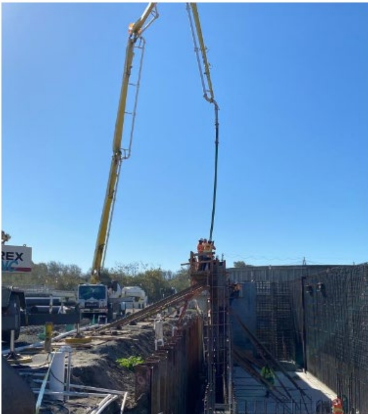
Placing Wall D_2021.11.05
