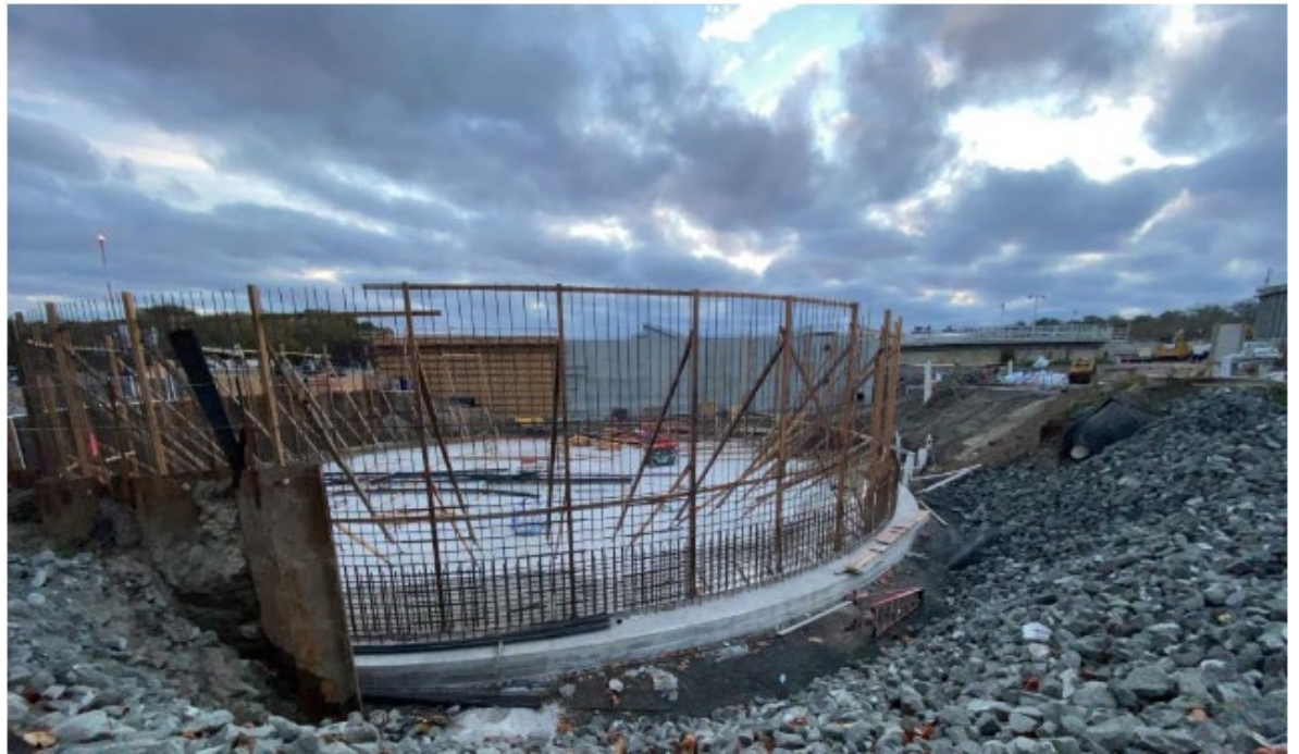
Secondary Clarifier No. 2 Rebar_2021.12.20
