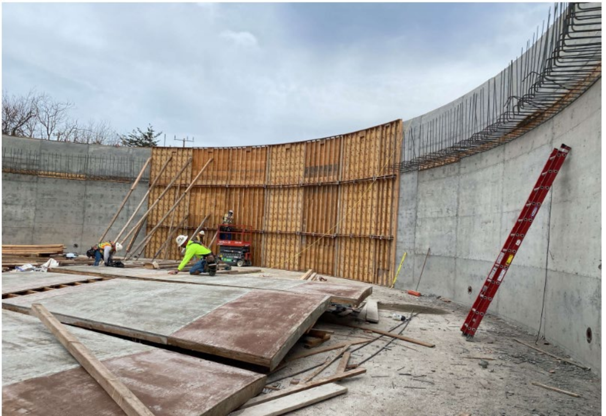
Secondary Clarifier No. 2 Formwork_2022.01.31
