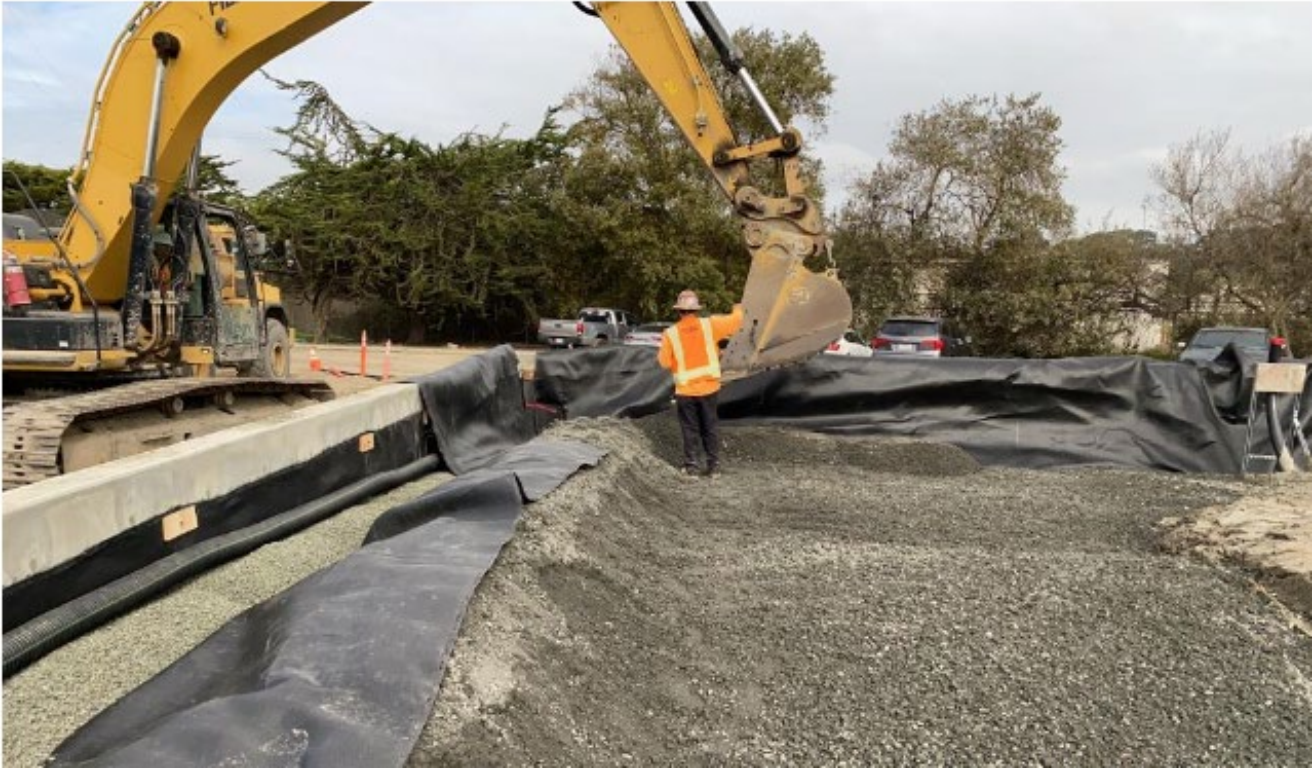
Blower Building Load Transfer Platform Installation_2021.12.14
