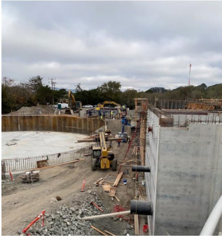
Formwork along the Aeration Basin_2021.12.03
