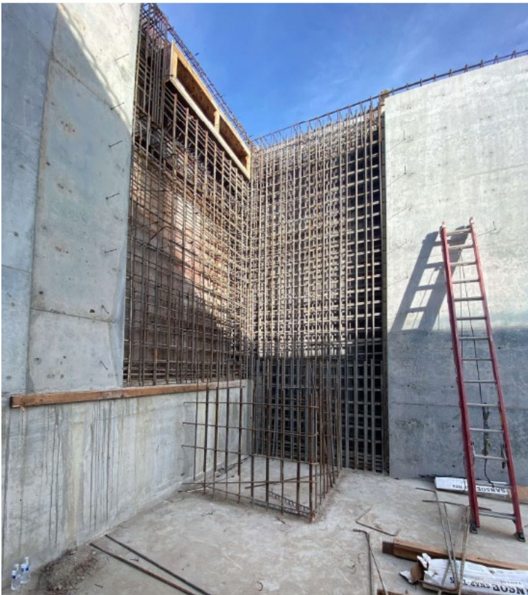
North Aeration Basin Wall Rebar_2022.01.10
