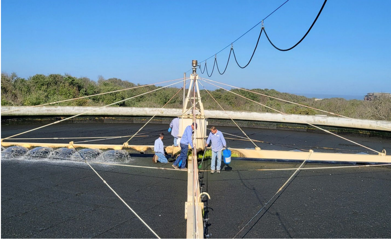
Billy Romhild, Mike Arias, Justin Musick and Rick Jackman performing monthly maintenance on the Fixed Film Reactor.
