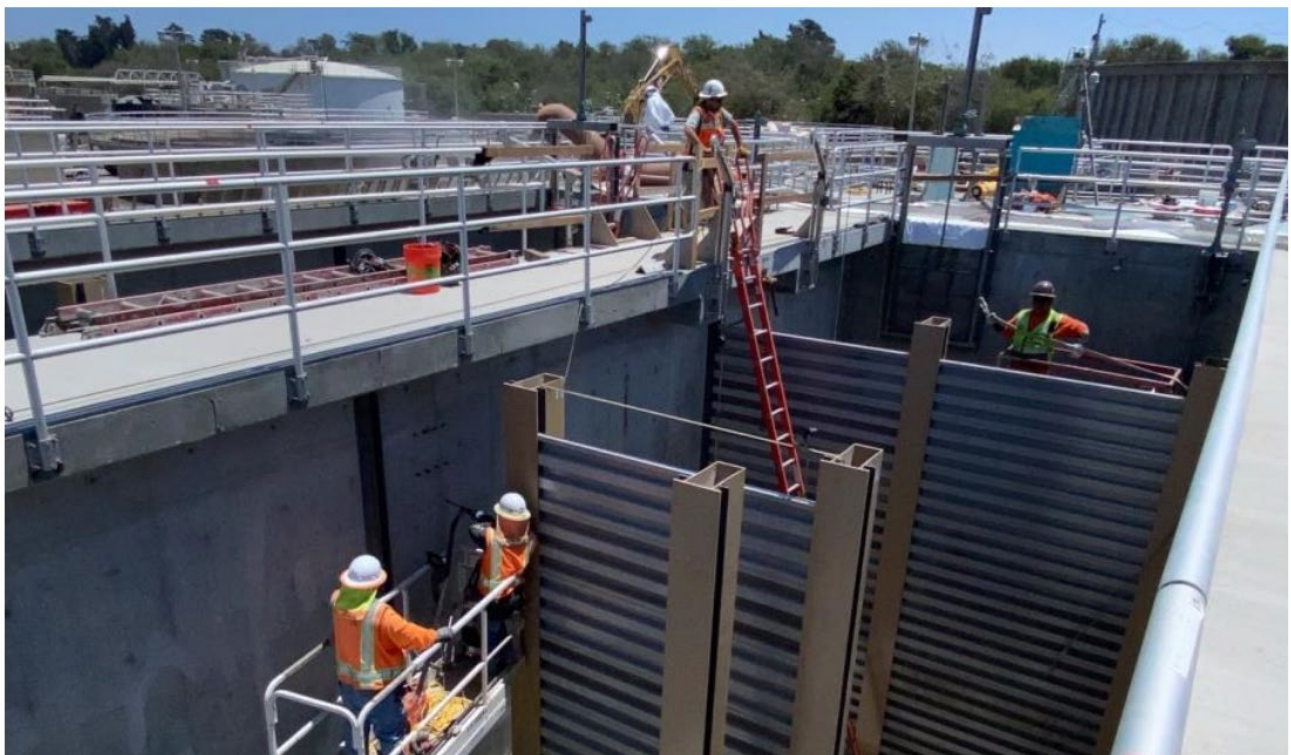
Aeration Basin Baffle Wall Installation_2022.06.21
