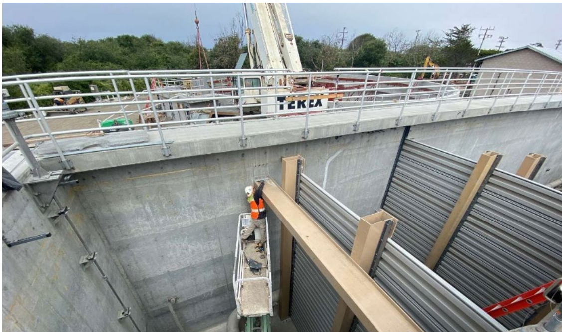
Aeration Basin Baffle Wall Installation_2022.07.05
