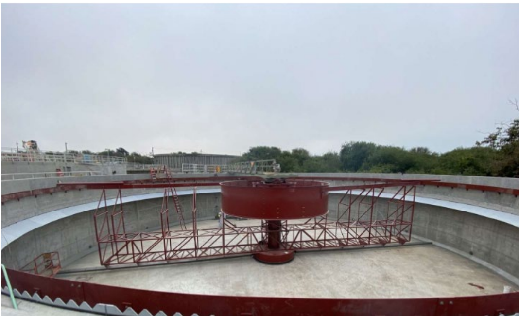
SC2 Lower Baffle Installed_2022.07.11
