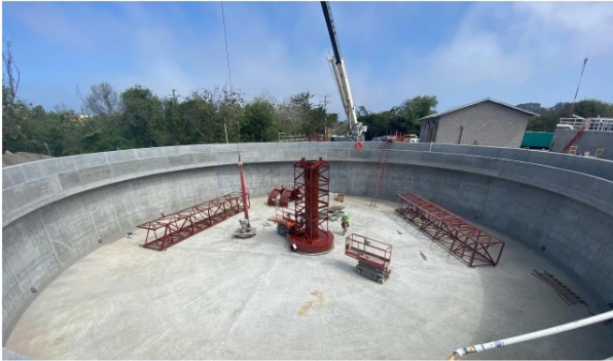
Secondary Clarifier No. 2 Progress_2022.05.24
