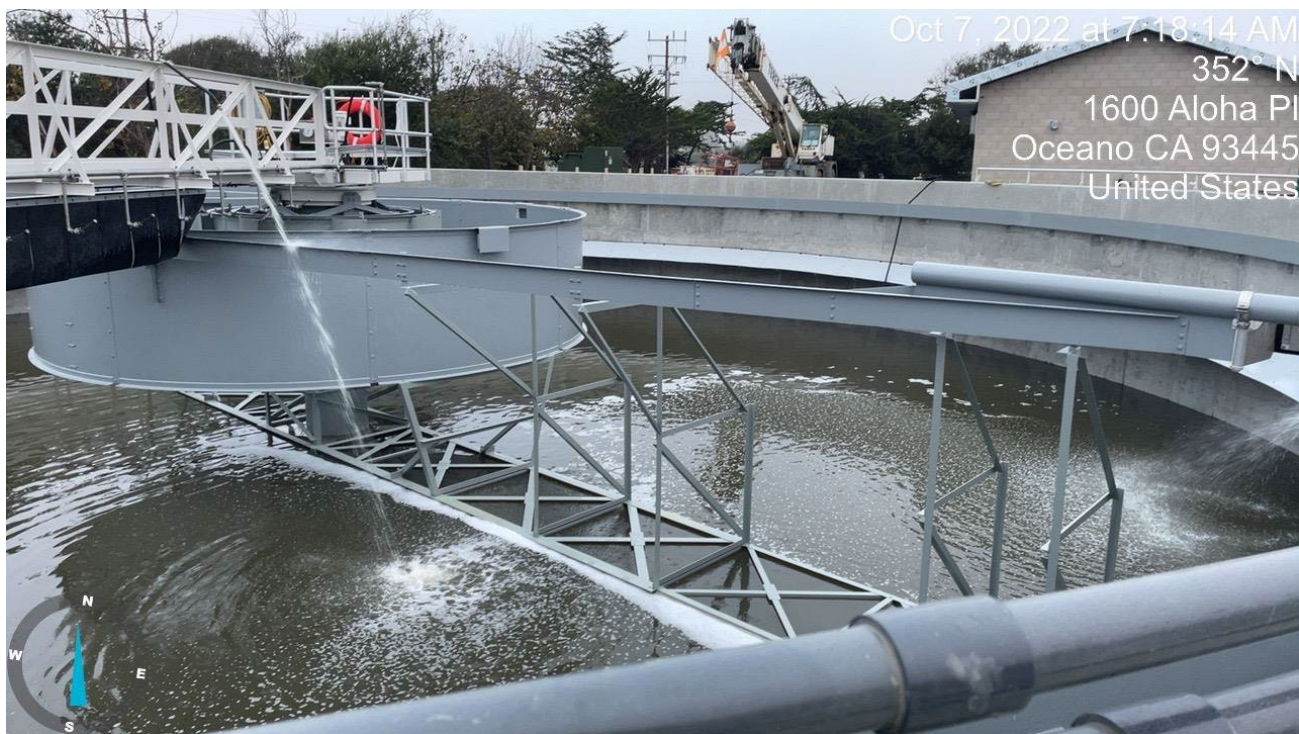
Filling Secondary Clarifier No. 2_2022.10.07
