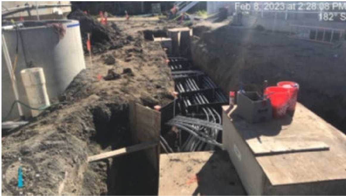
Electrical Ductbank EHH/SHH 11 to 12_2.8.2023
