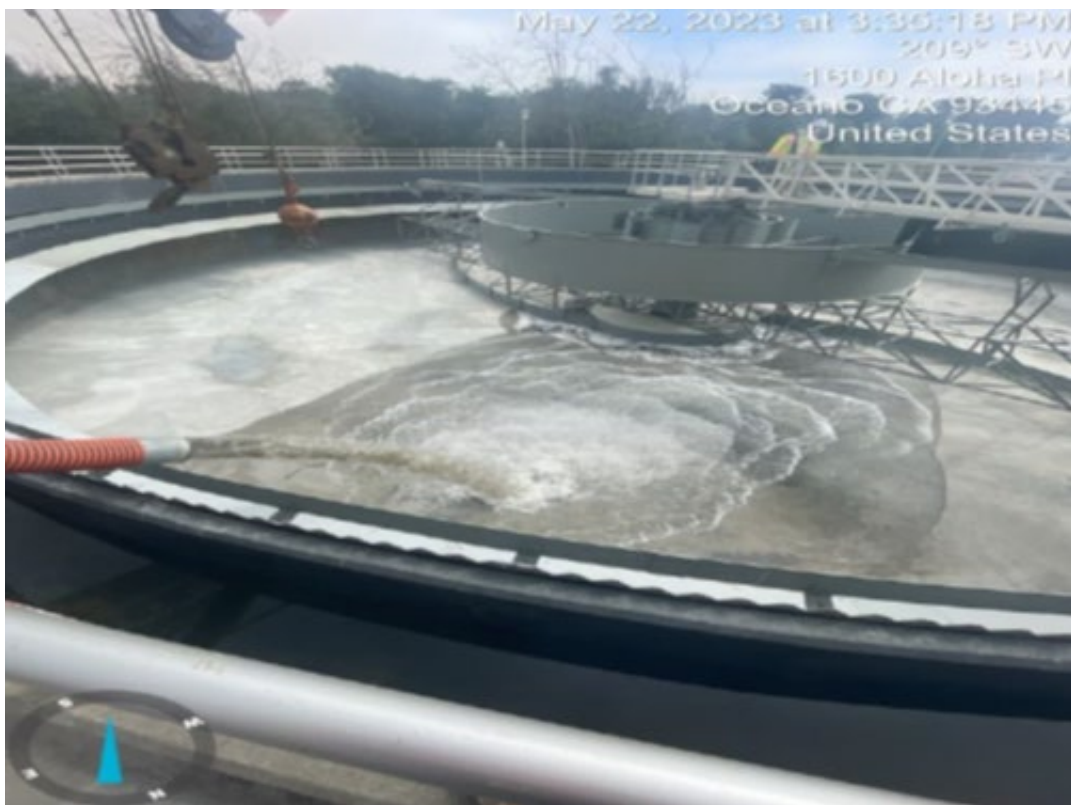
Filling Secondary Clarifier No. 1_5.22.2023
