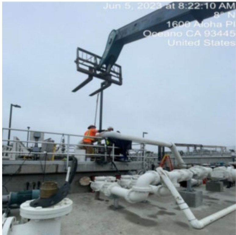
Temporary Piping for RAS Pump Testing at SC 2_6.5.2023
