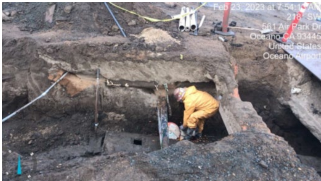
Sawcutting 30-inch Abandoned Pipe_2.23.2023
