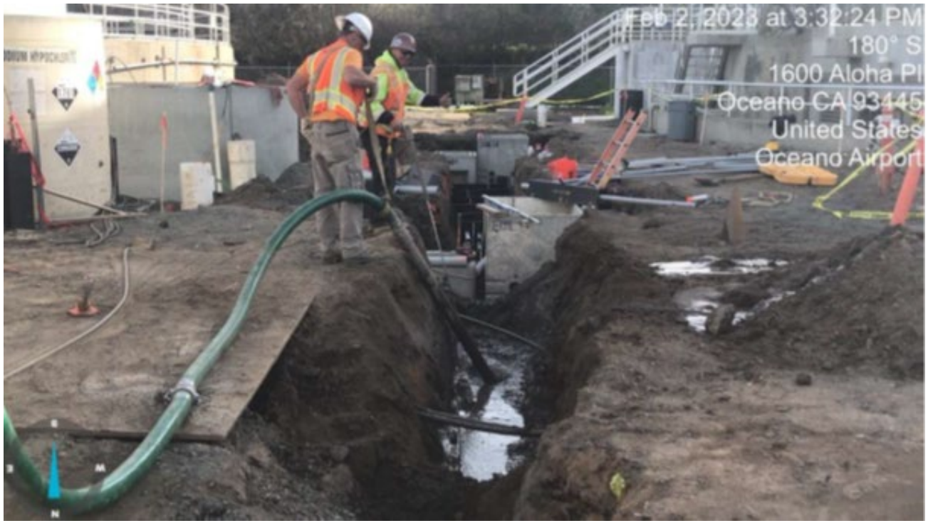
Ductbank Excavation_2.2.2023
