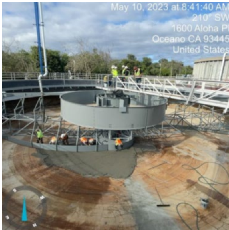
Secondary Clarifier No. 1 Grout_5.10.2023
