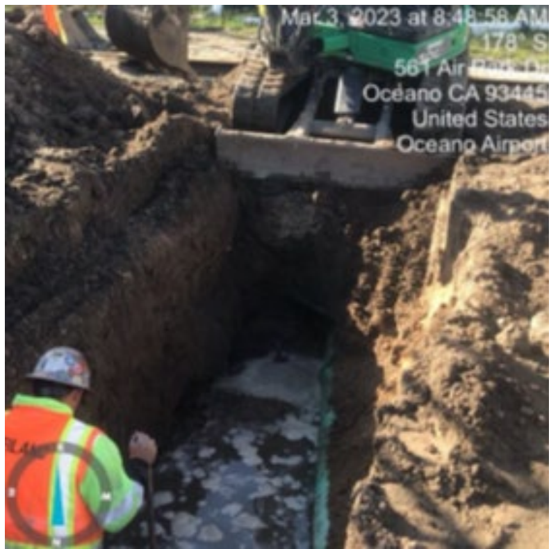
Excavating for Storm Drain_3.3.2023
