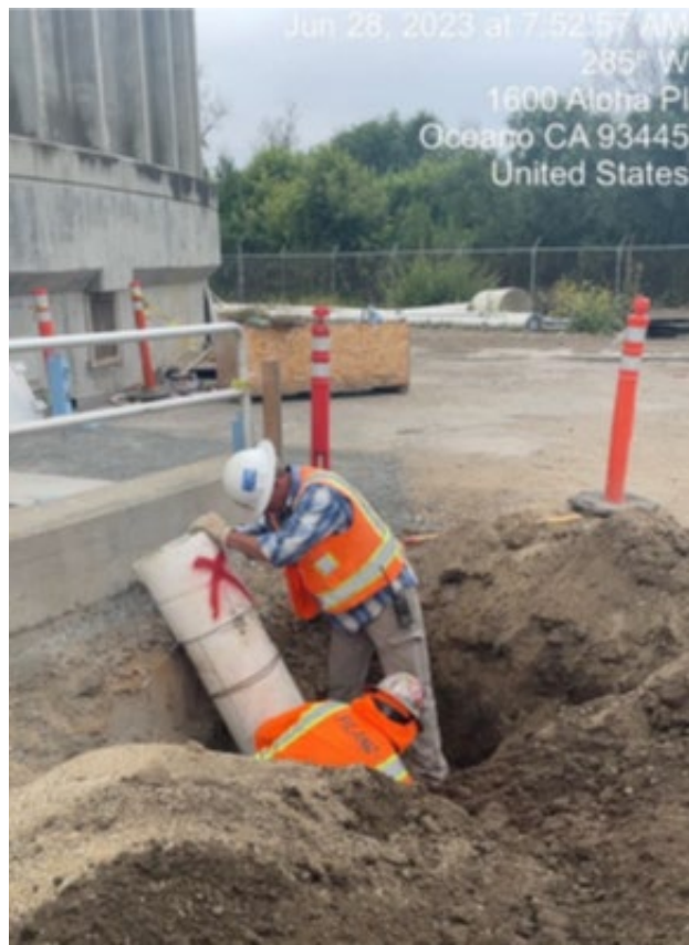
Dewatering Well Abandonment_6.28.2023
