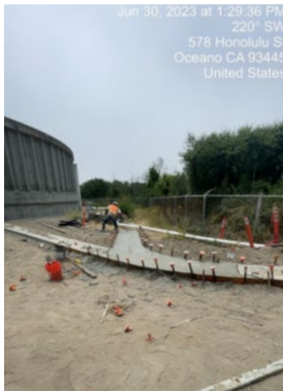
Curb and Gutter Placement_6.30.2023
