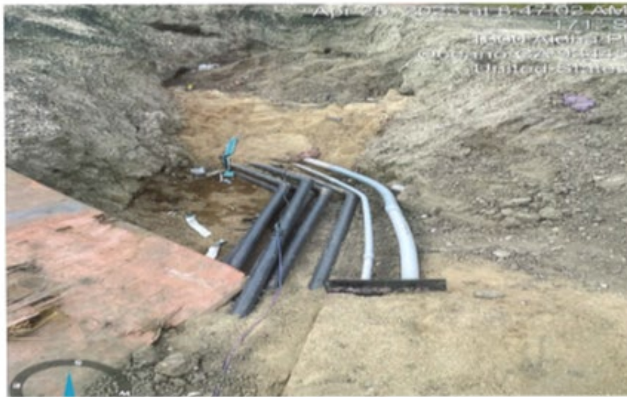
Repair of Damaged Conduits and Conductors for FFRE_4.21.2023
