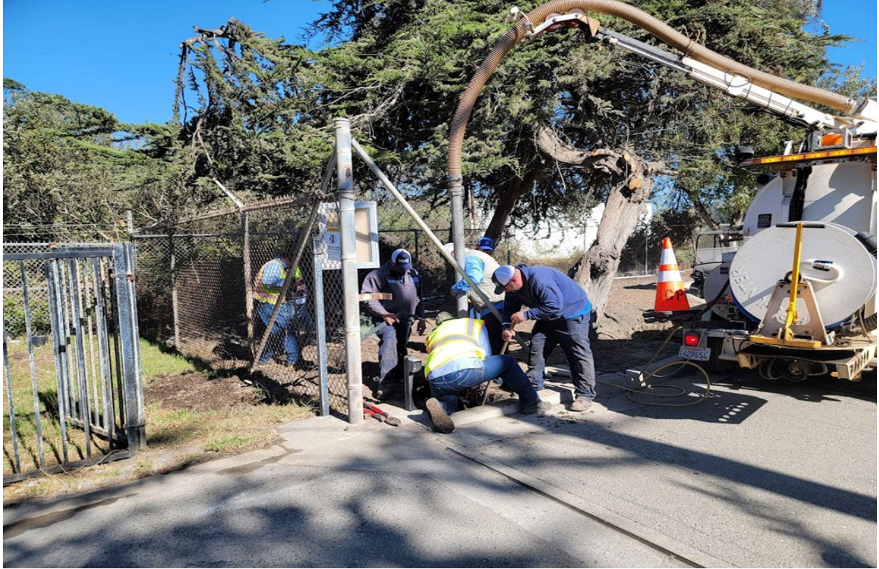
OCSD Crew assisting District Plant Operators with locating a leaking water line.
