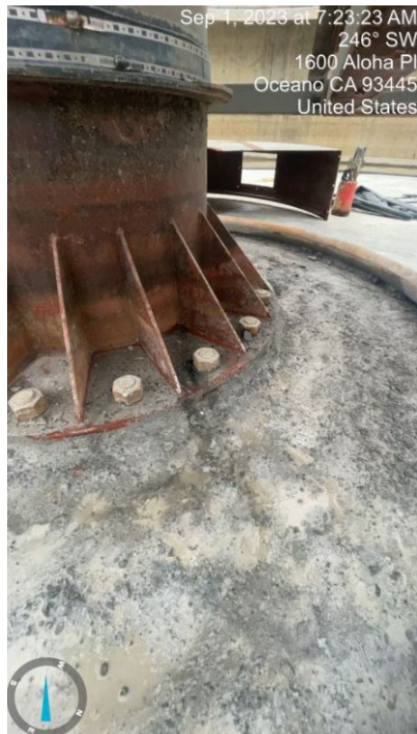
9.1.23. Leaking Bolt
