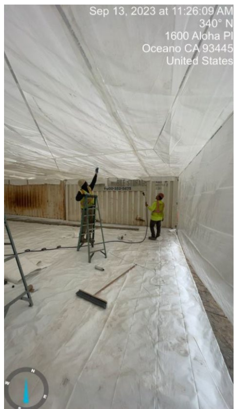
9.13.23 PC1 Mechanism Coating Containment
