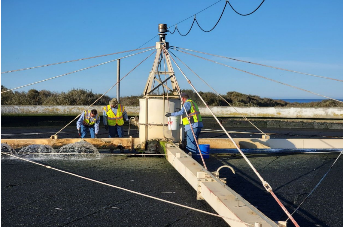
Plant Operations staff performing a monthly fixed film reactor oil sample, orifice and net cleaning, and the replacement of a broken orifice.
