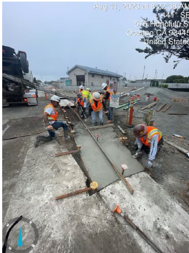
8.11.23 Curb & Gutter Concrete Placement
