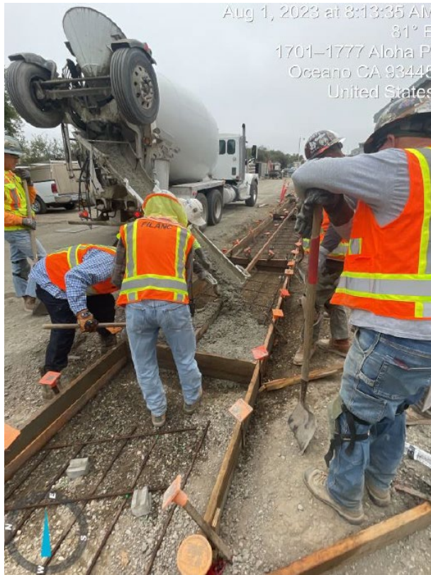
8.1.23. Concrete Curb & Gutter Placement
