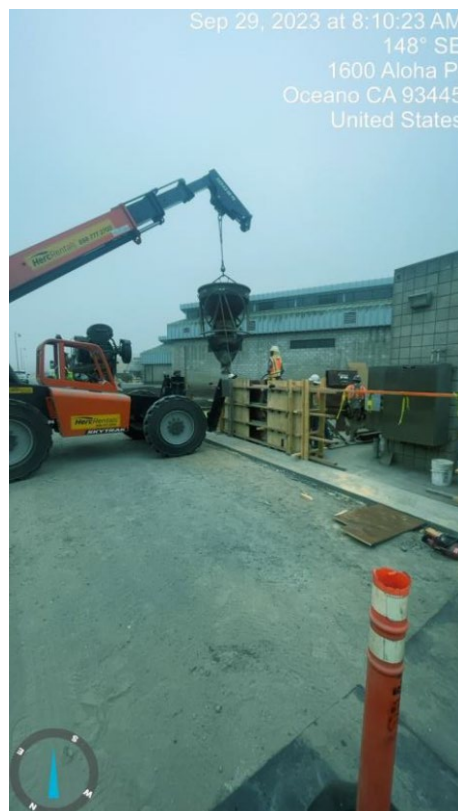
9.29.23 Generator Floodwall Concrete Placement
