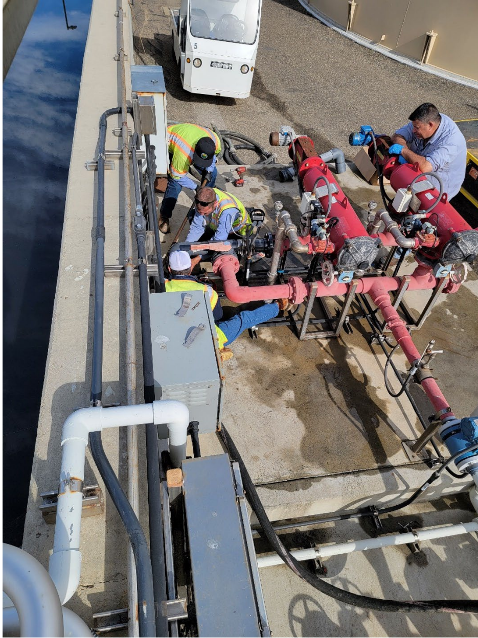
Operations staff performing the installation of the new Amiad reclaim water filtration piping. (Operators Pictured: Mike Arias, Billy Romhild, Justin Musick, and Nick Kurokawa)
