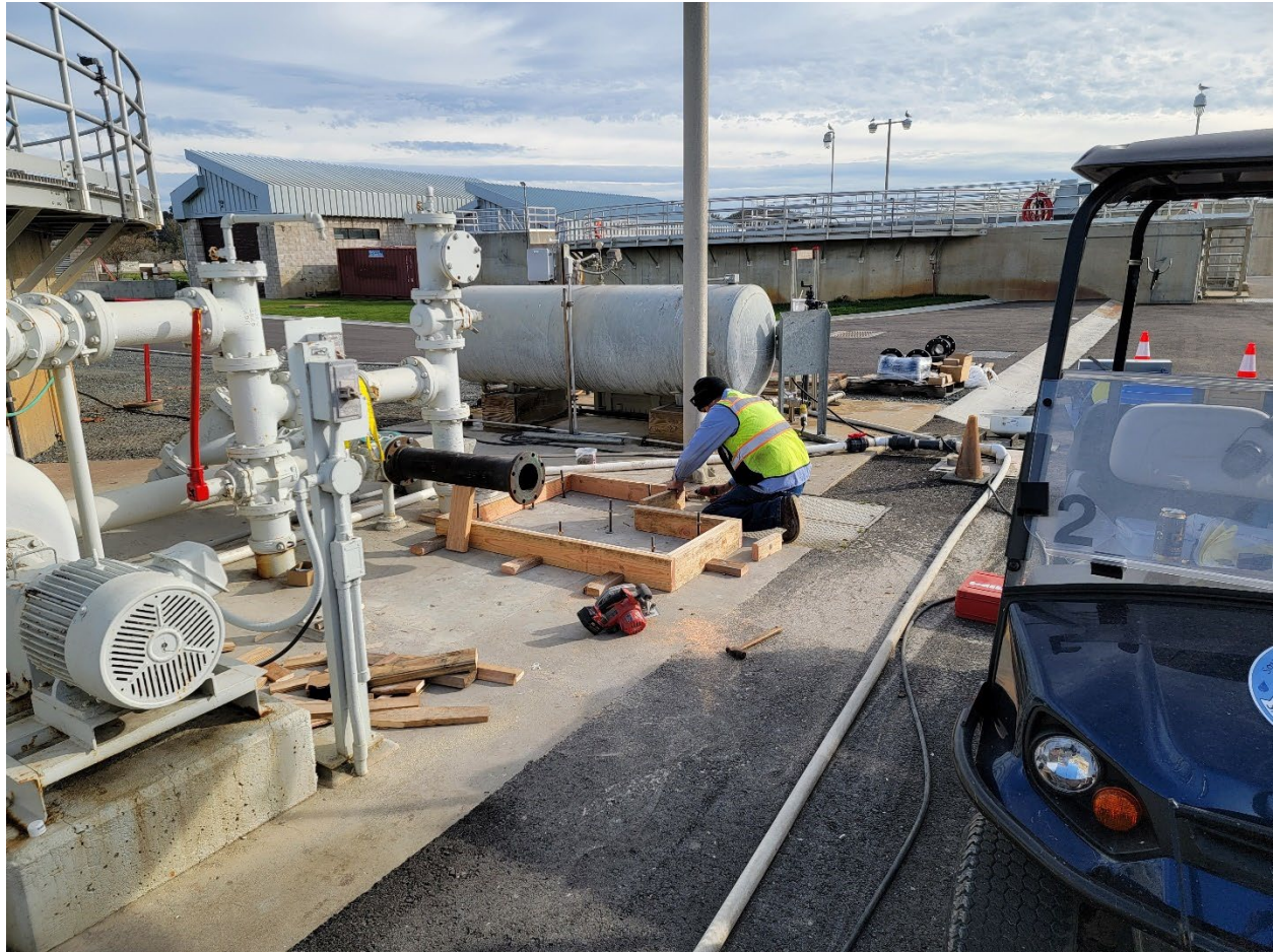
Operator Justin Musick installing forms for new PC2 sludge pump installation.
