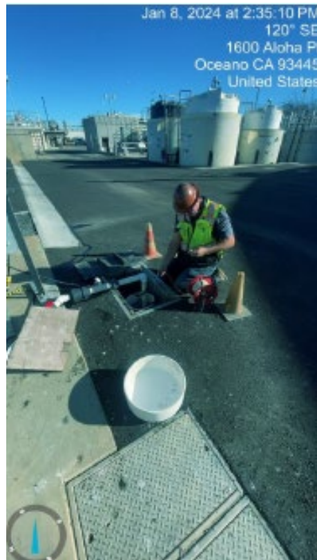
1.8.24. Dewatering Well Maintenance
