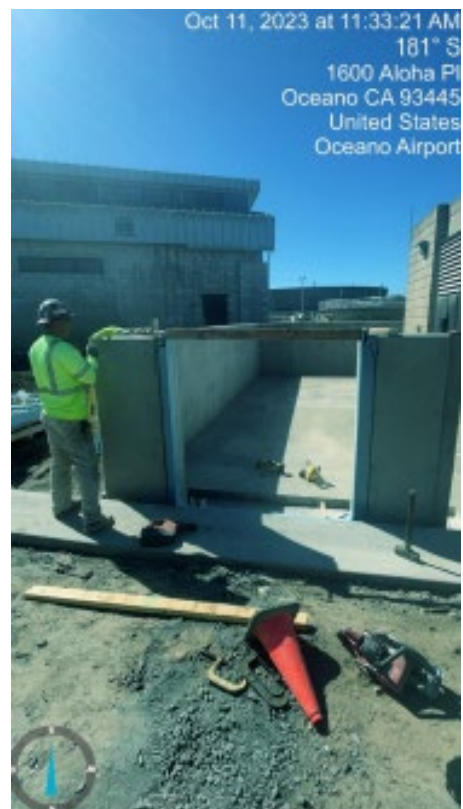
10.11.23 Generator Floodwall Frame
