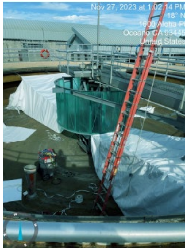
11.27.23 Primary Clarifier No.1 Mechanism Coating
