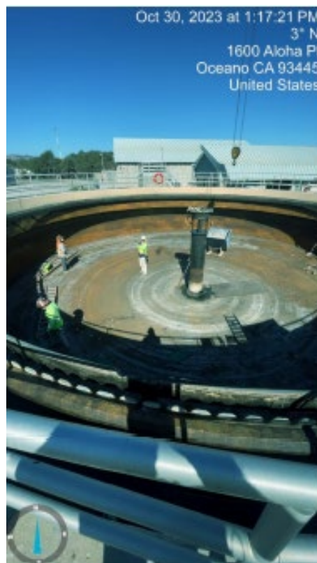
10.30.23 PC1 Mechanism Removal
