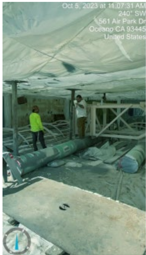
10.3.23 Coating PC1 Mechanism Components
