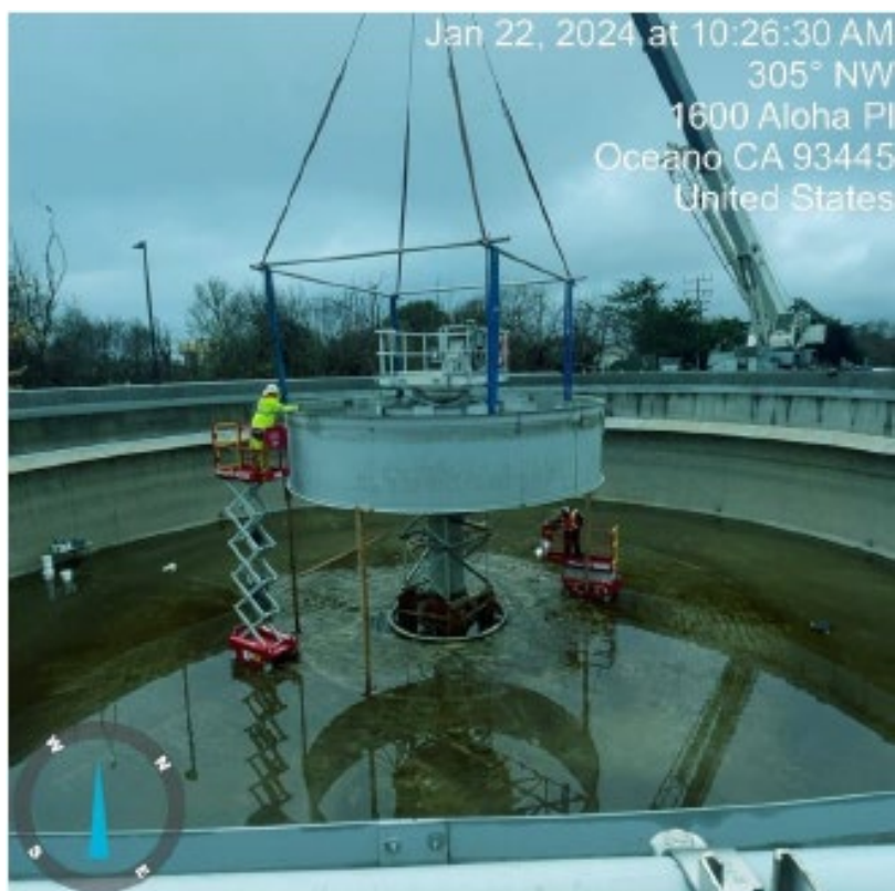
1.22.24. SC2 Mechanism Removal
