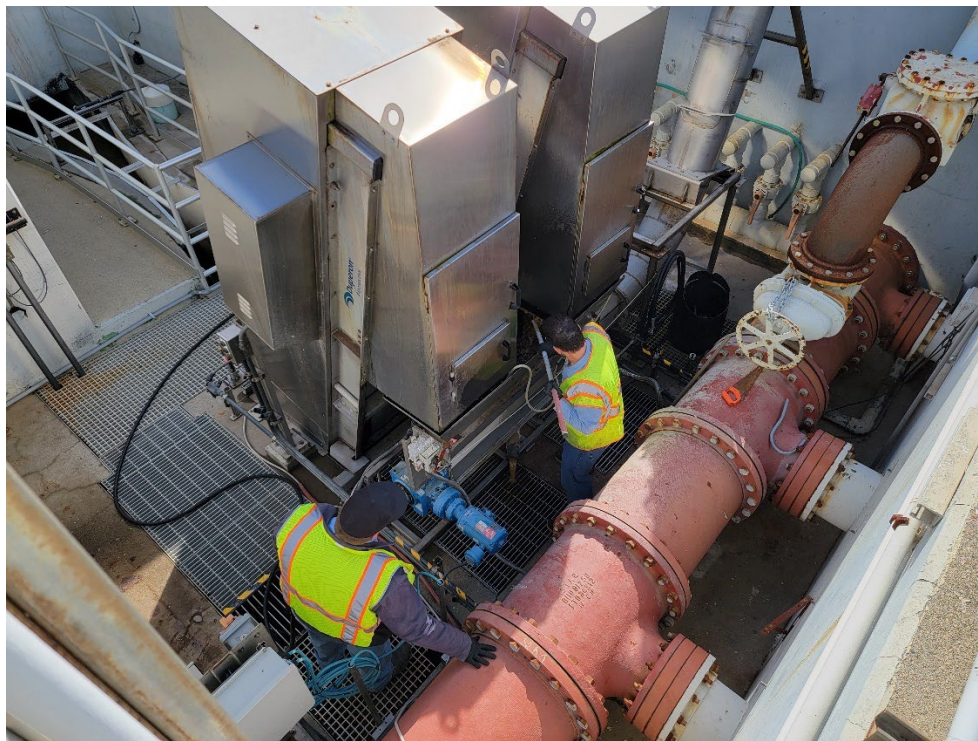
Operator Chris Rigoni providing some overwatch of Operator in Training Robert Grajeda while he is clearing a blockage in the District's mechanical bar screens.
