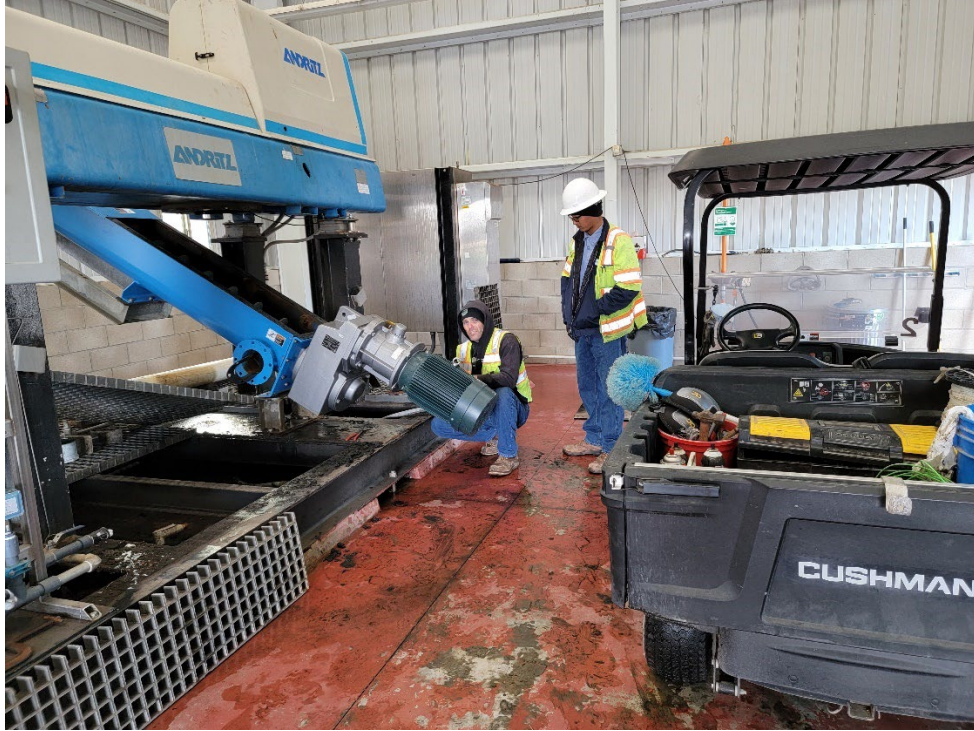
Operator Justin Musick and Operator in Training Nick Kurokawa installing electrical on new centrifuge auger motor.
