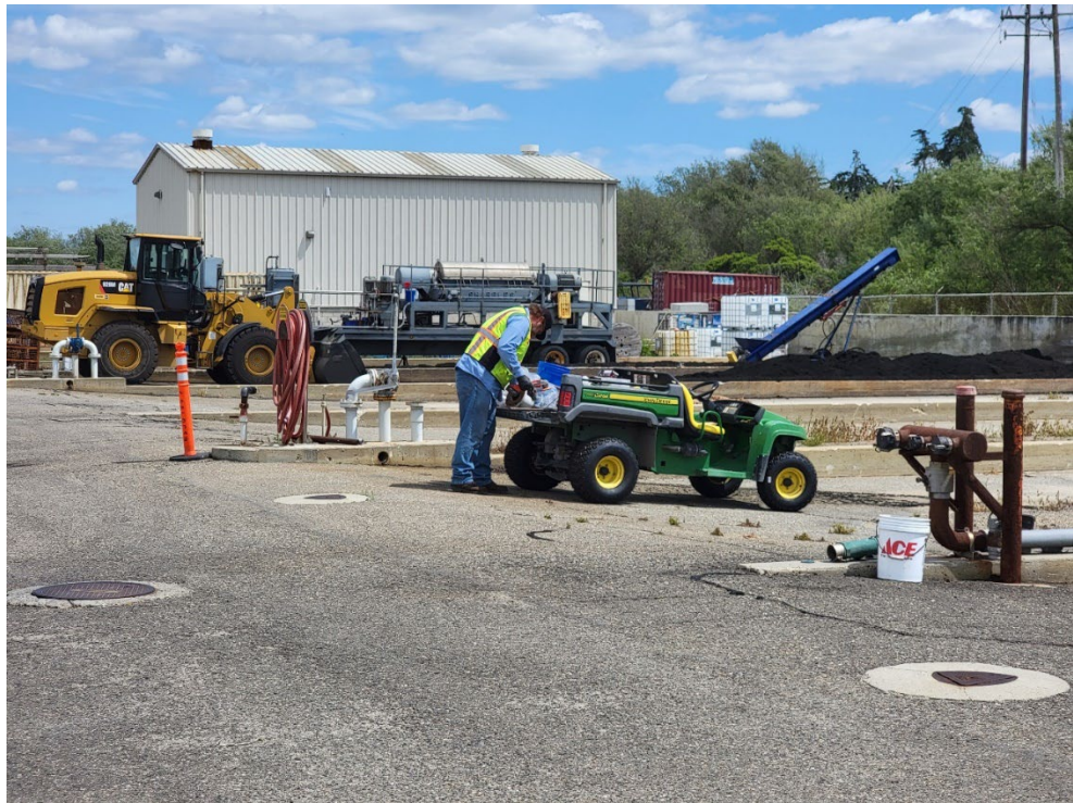
Operator Chris Rigoni installing new sludge bed valves.
