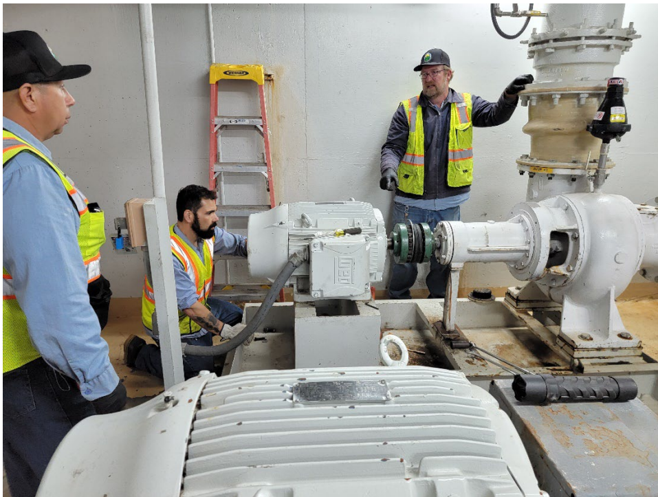
Operators in Training Everardo Vargas and Robert Grajeda receive training from Operator Chris Rigoni in the removal of Influent Pump No. 3.
