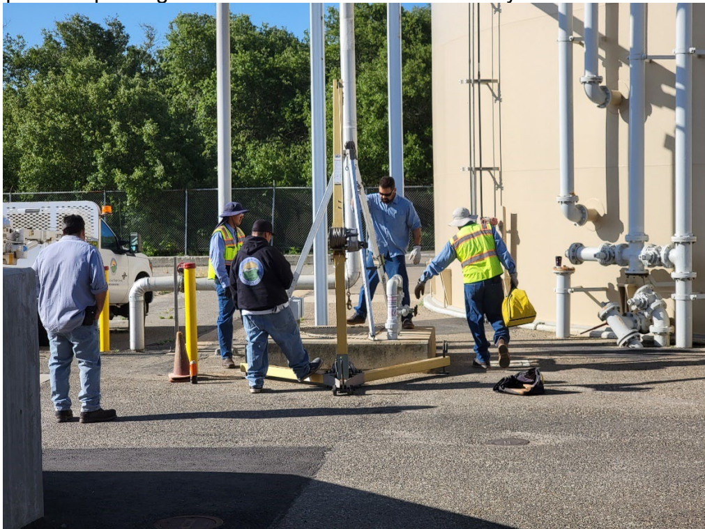
District Operators in Training being trained on the setup of the davit crane and tripod.
