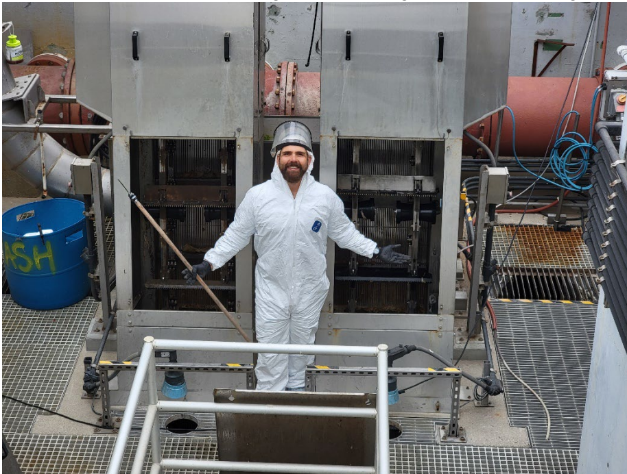
District Operator in Training/Intern Robert Grajeda showing off the difference between a dirty mechanical bar screen and a freshly power washed mechanical bar screen.
