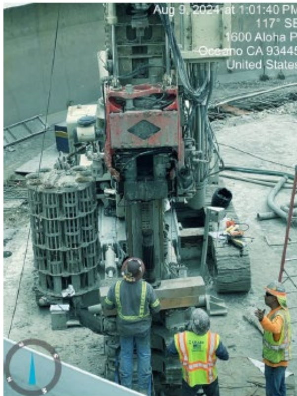
8.9.24 Reassembling Drill Rig
