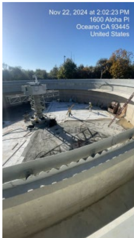
11.22.24 Concrete Placement Quadrant #3 Curing Blankets
