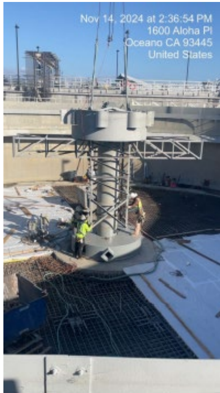
11.14.24 SC2 Mechanism Re-Assembly
