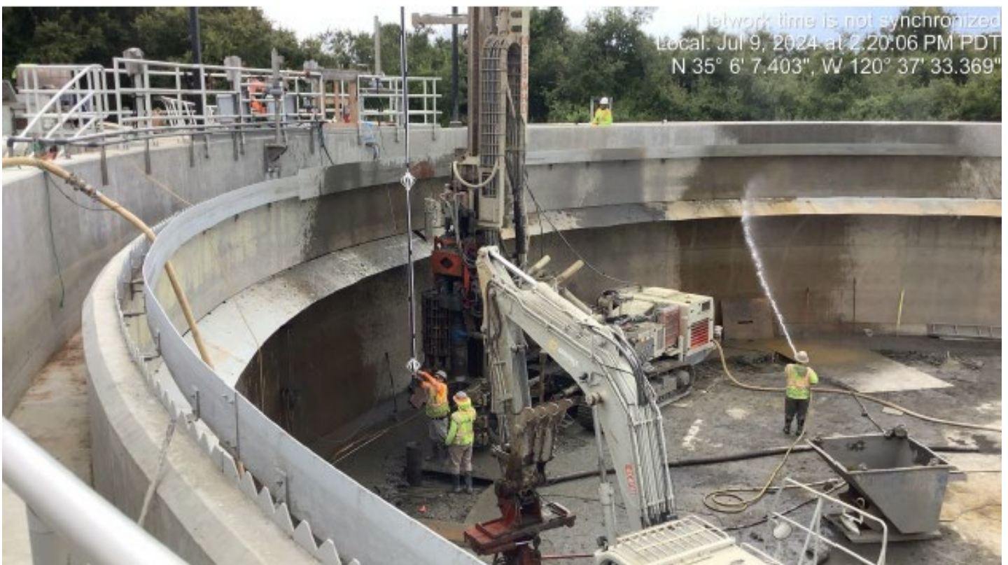
7.9.24 Micropile Tie-Rod Installation
