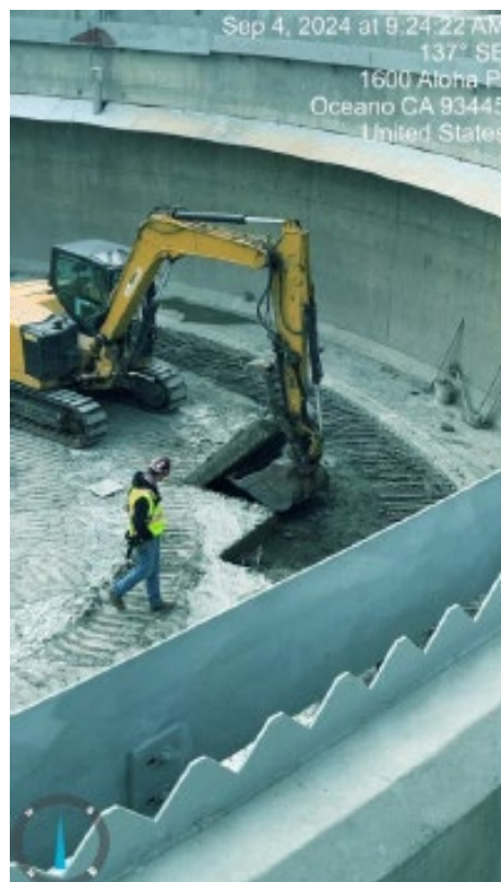
9.4.24 Demolition of the SC2 Slab Begins
