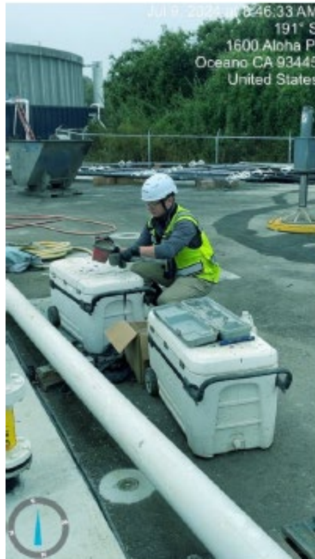
7.9.24 Grout Quality Control
