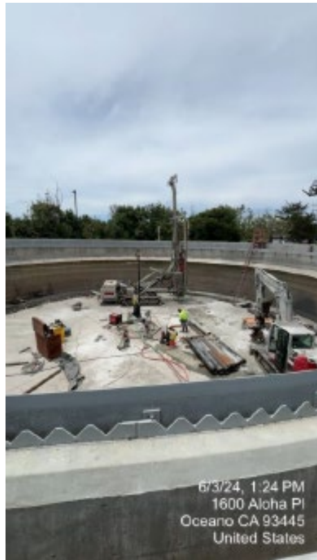
6.3.24 Concrete Coring
