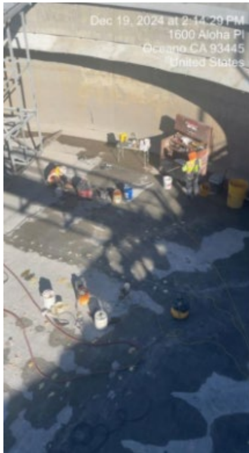
12.19.24 SC2 Concrete Crack Injection
