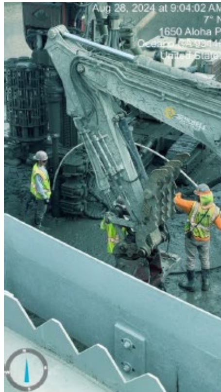
8.28.24 Grouting a Micropile
