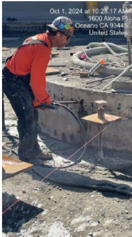
10.1.24 Concrete Coring to Obtain Depth
