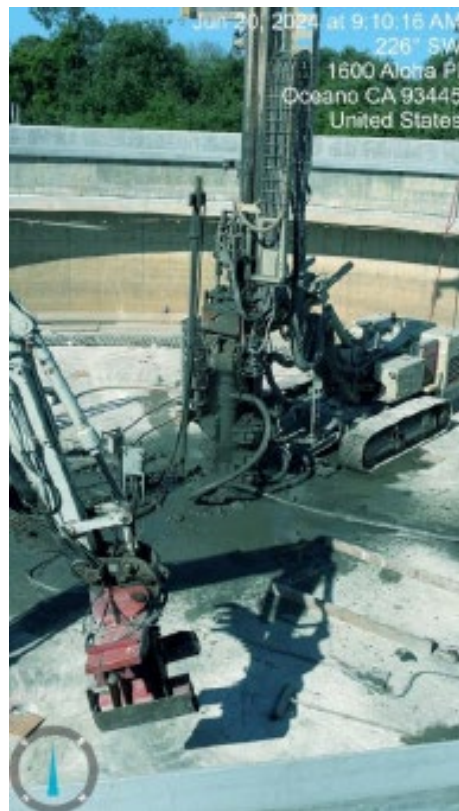
6.20.24 Micropile Drilling
