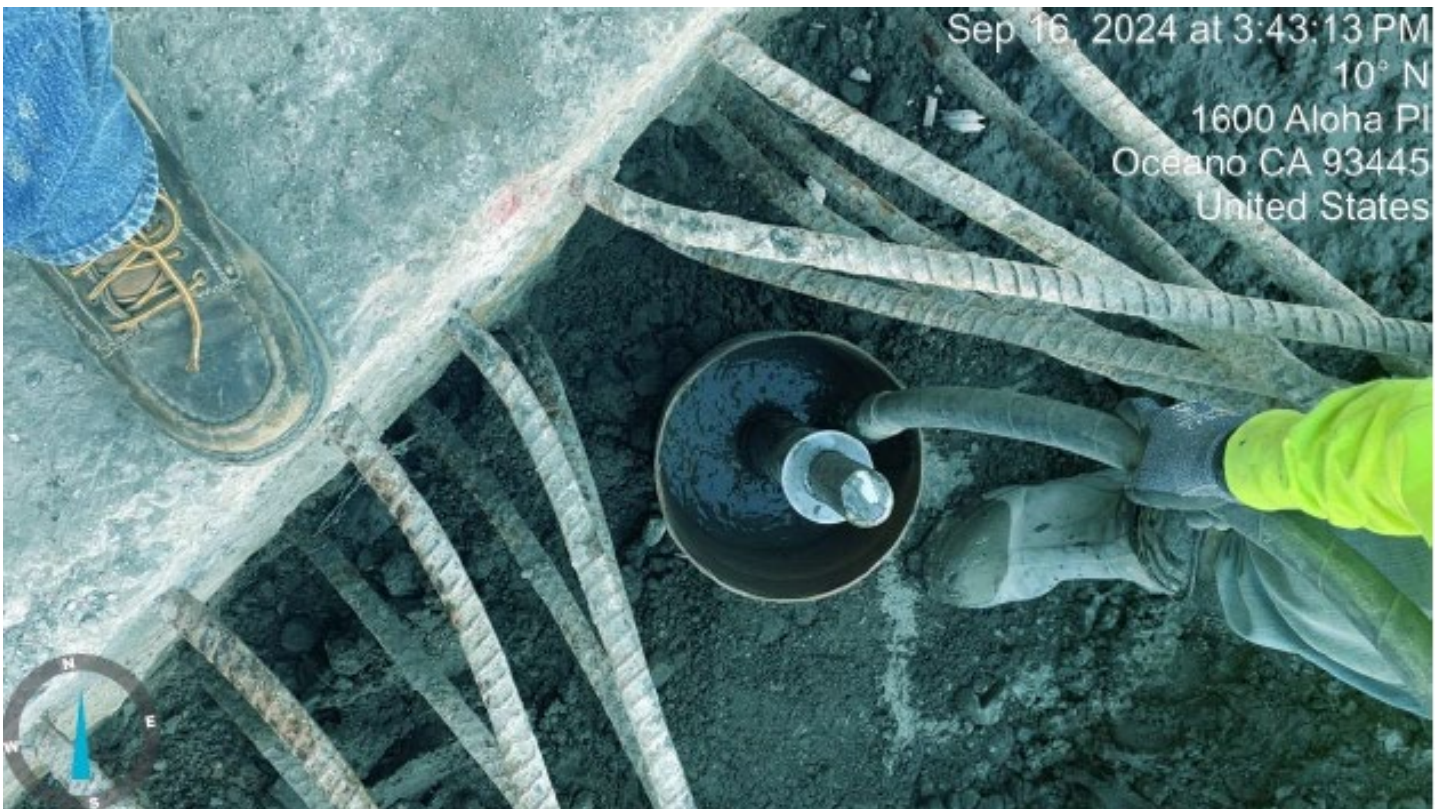
9.16.24 Micropile Grout
