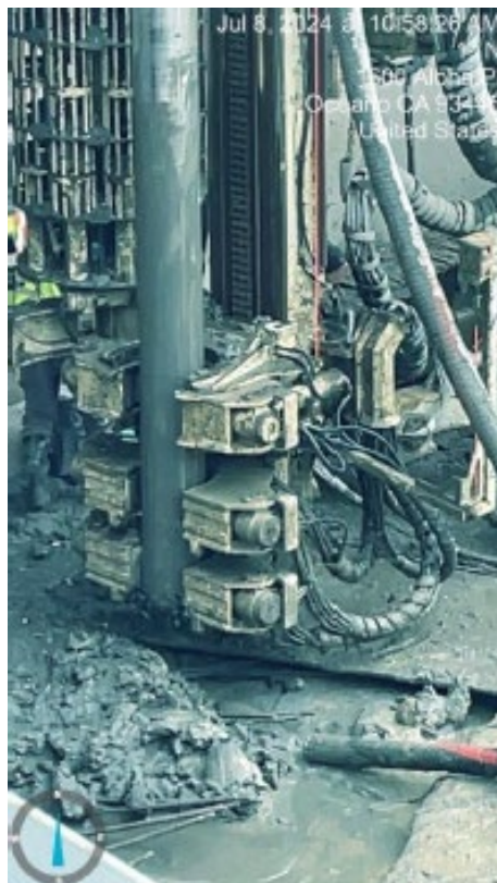
7.8.24 Micropile Installation Continued
