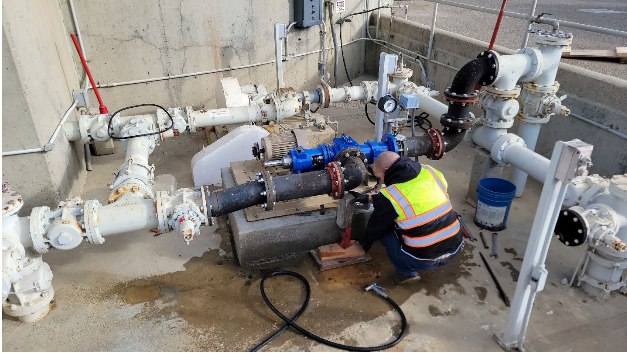
Operator Justin Musick installing new Primary Clarifier No. 1 sludge pump.
