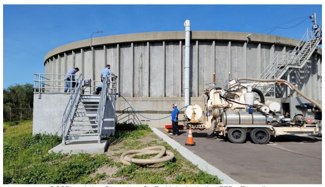
OCSD assisting Operations Staff with hydro-jetting FFR effluent line.
