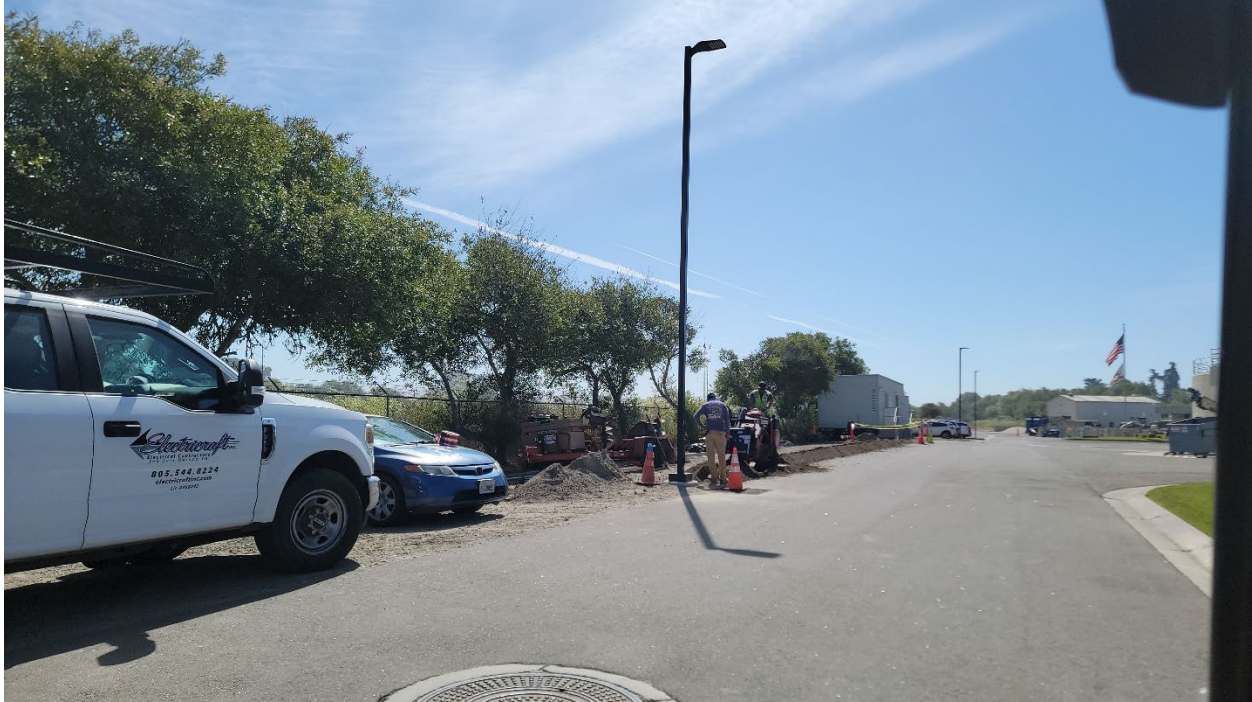
Electricraft trenching to install electrical conduit for Plant Light Replacement Project.
