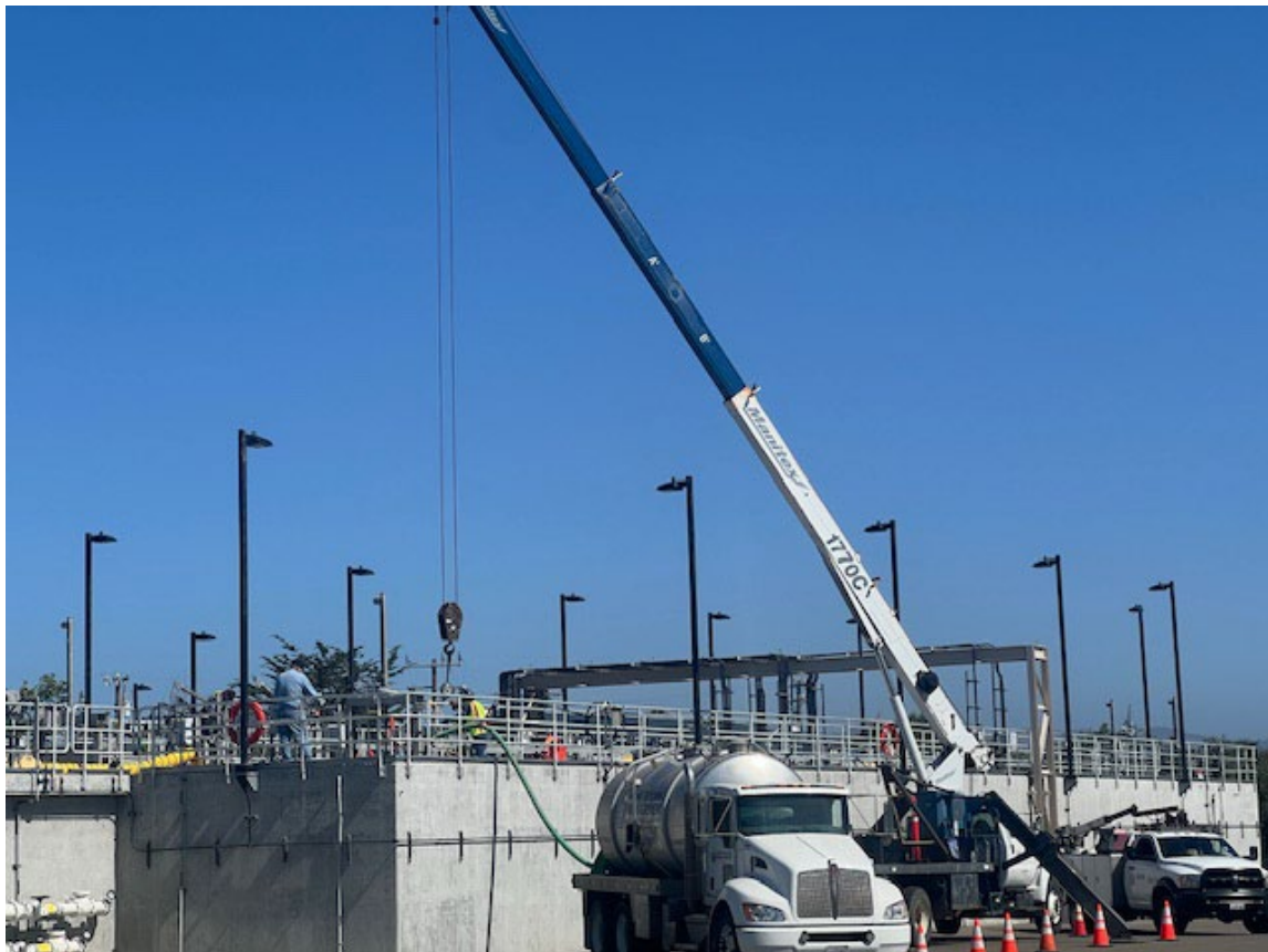
Fluid Resource Management performing the cleanout of Aeration Basin No. 2.
