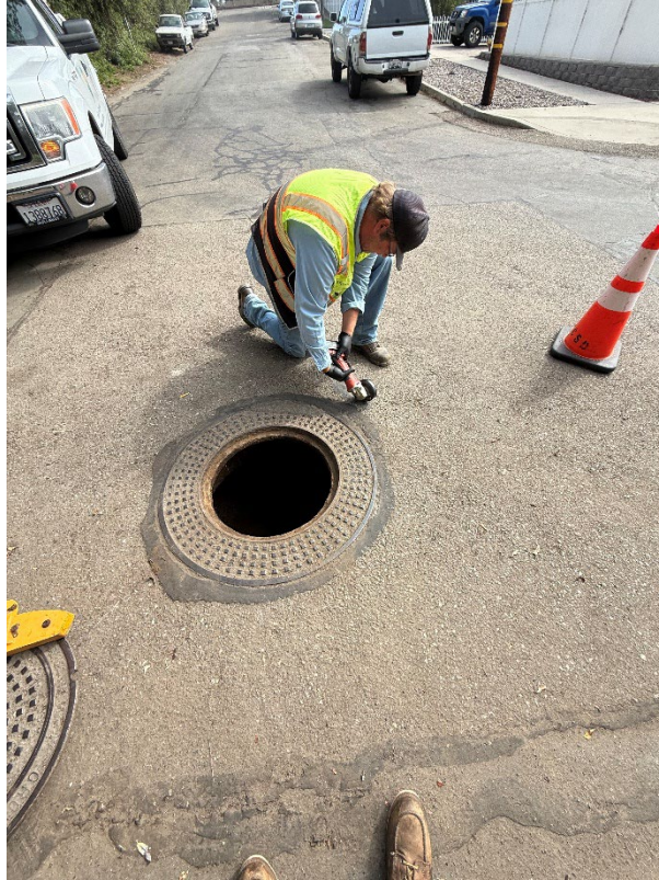
Senior Operator Christopher Rigoni performing installation of new float level system at a District manhole.
