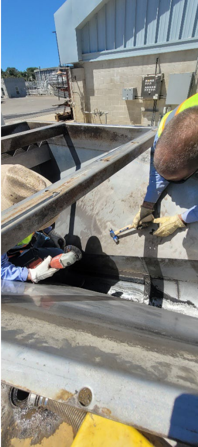
Operators Everardo Vargas and Justin Musick removing the Grit King classifier interior lining.
