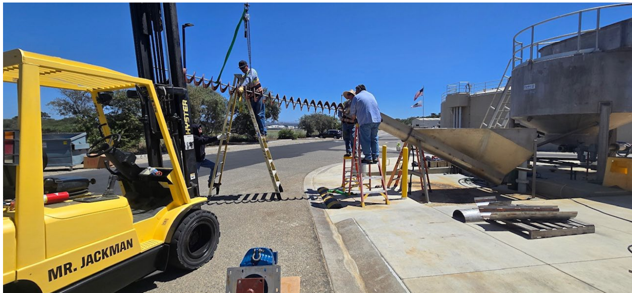
Operations Supervisor Mike Arias and Operators Justin Musick and Everardo Vargas installing the new Grit King classifier auger.
