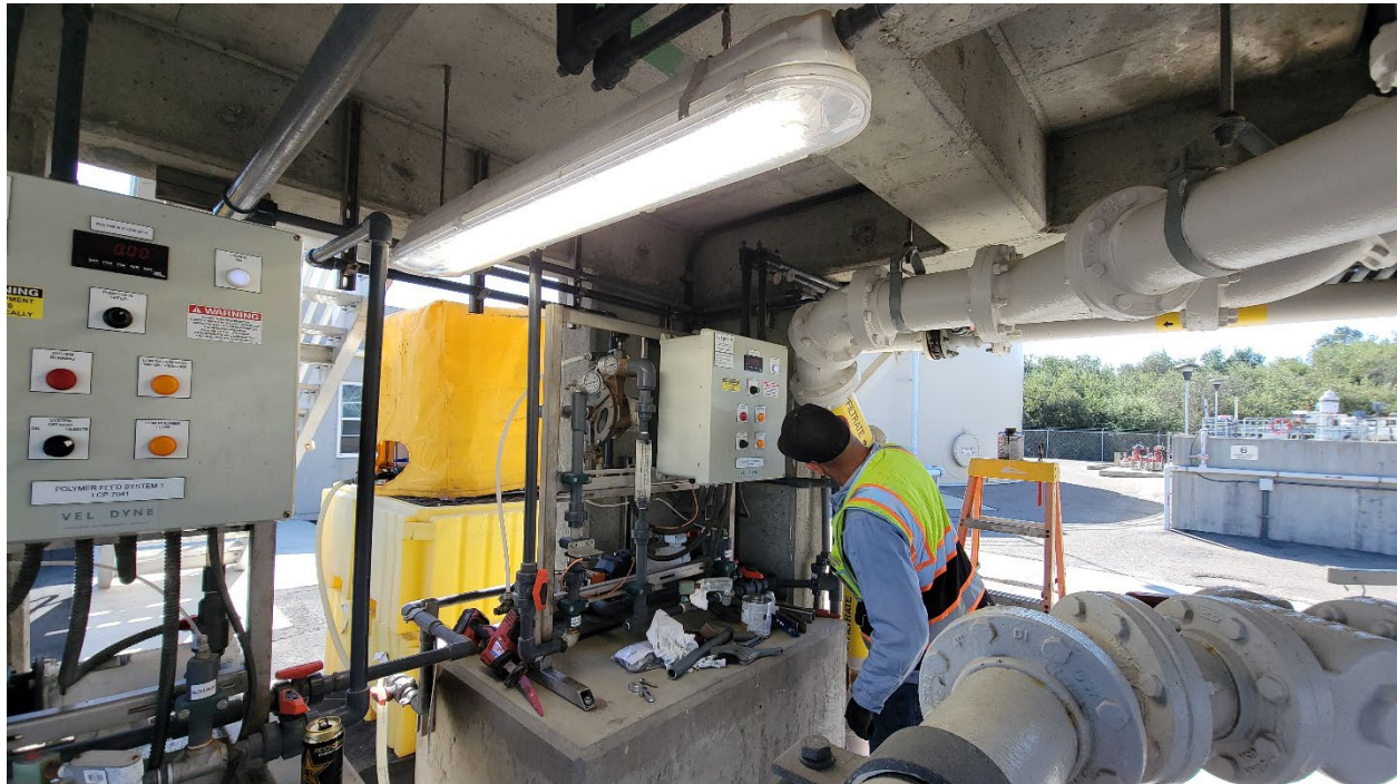
Operator Justin Musick installing new reclaim water line to RDT polymer system.
