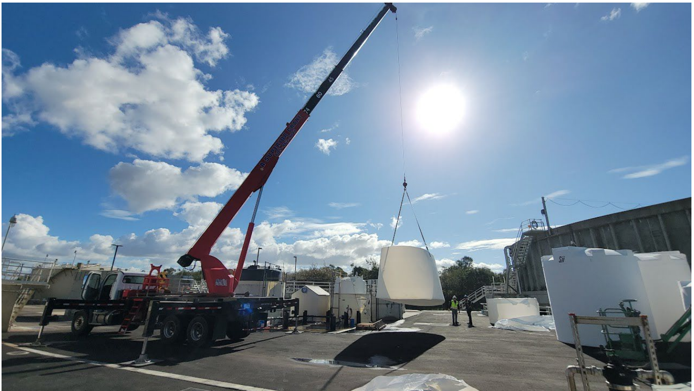
Installation of new chemical tanks.
