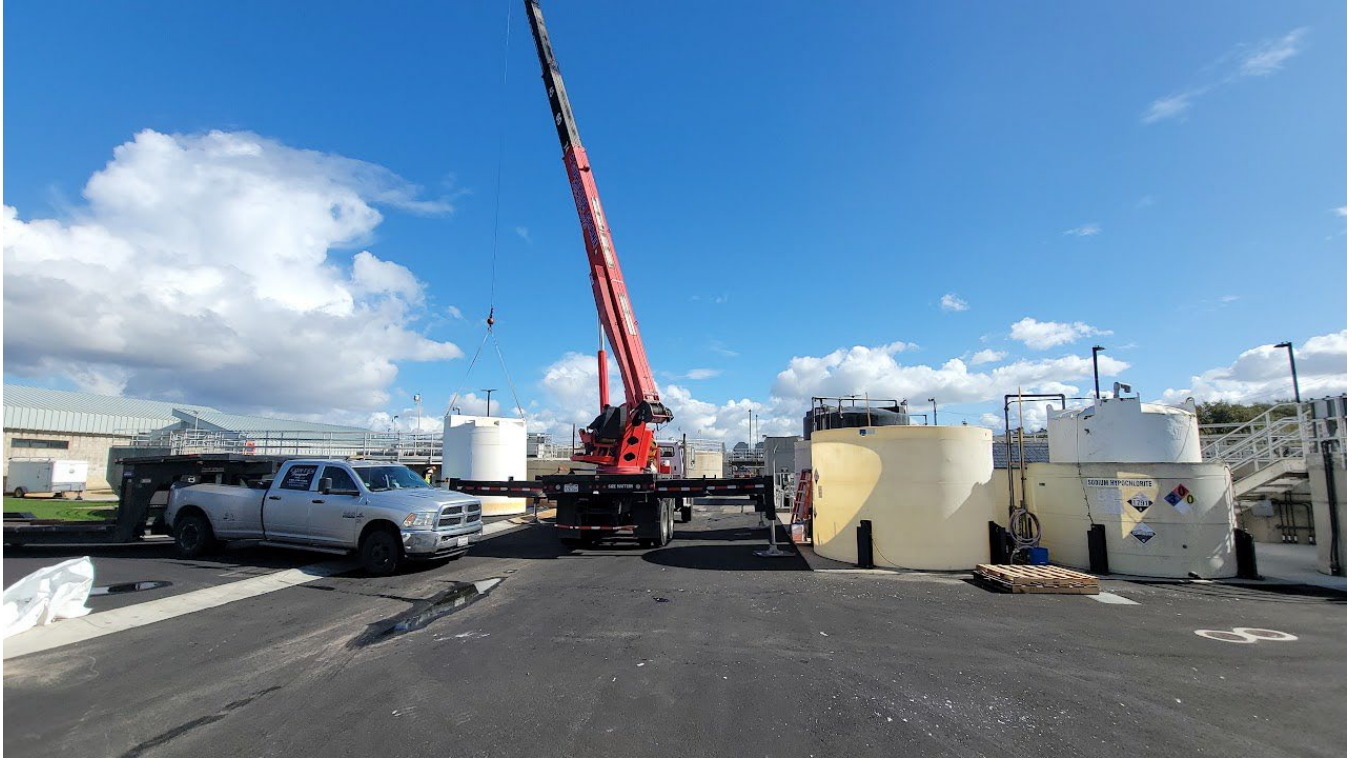
Removal of old chemical tanks.
