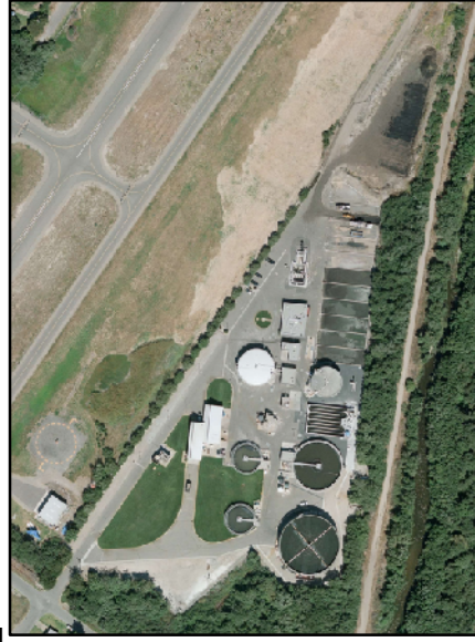
SSLOCSD Wastewater Treatment Plant
