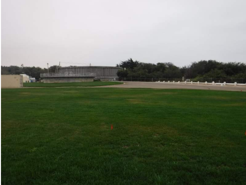
Photo 7 - South toward new Secondary Clarifier and new Aeration Basin
