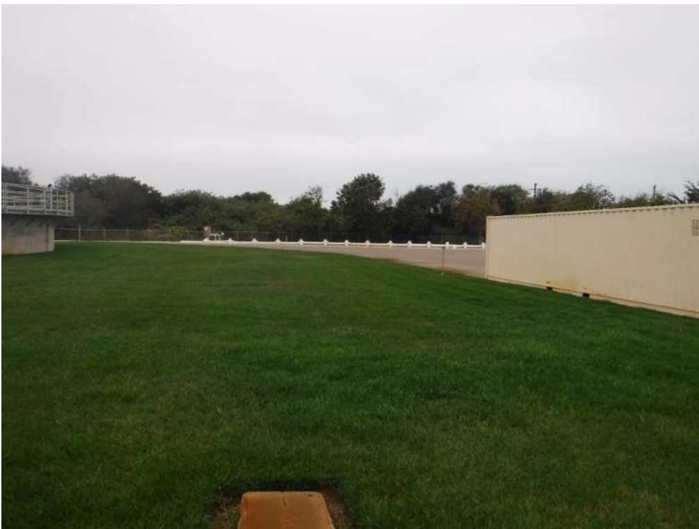
Photo 12 - West toward new Aeration Basin (south of road)
