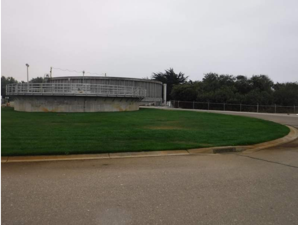
Photo 5 - West (slight south) toward new Secondary Clarifier
