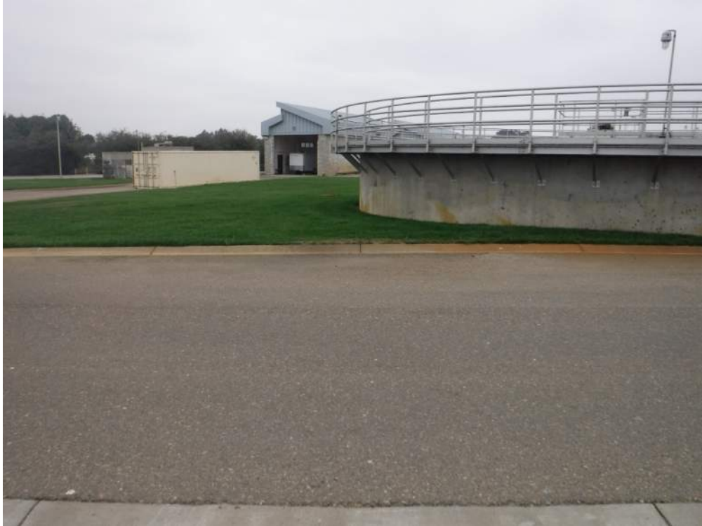
Photo 15 - East (new Aeration Basin on left side of photo)
