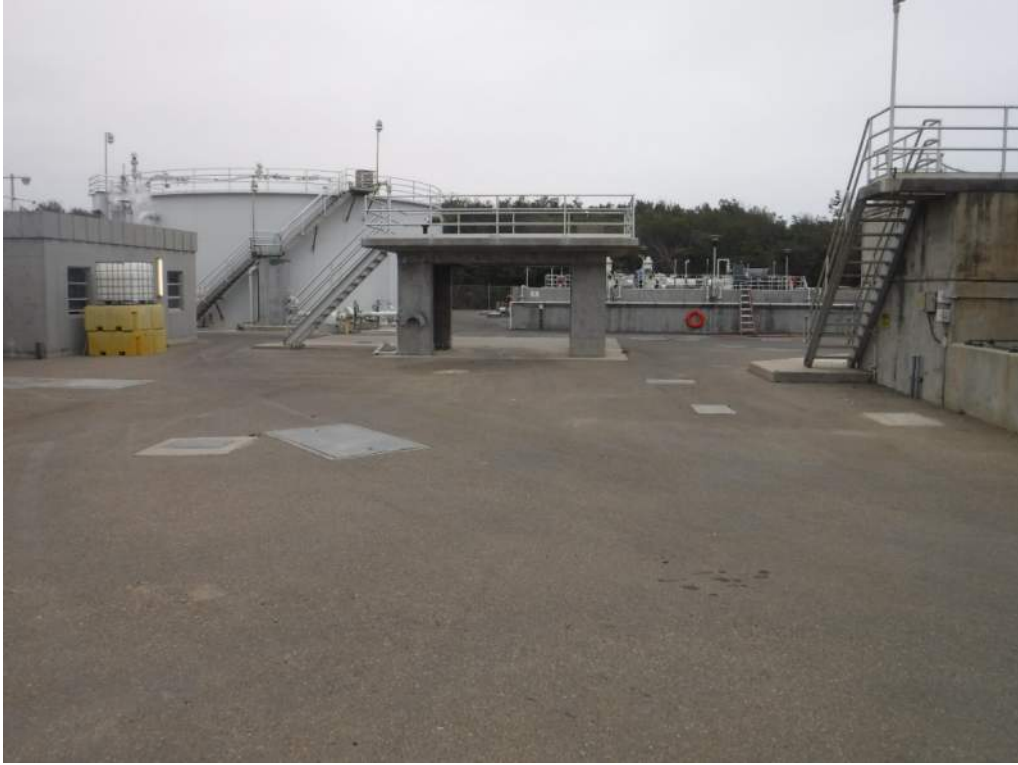
Photo 17 - South toward new Centrifuge
