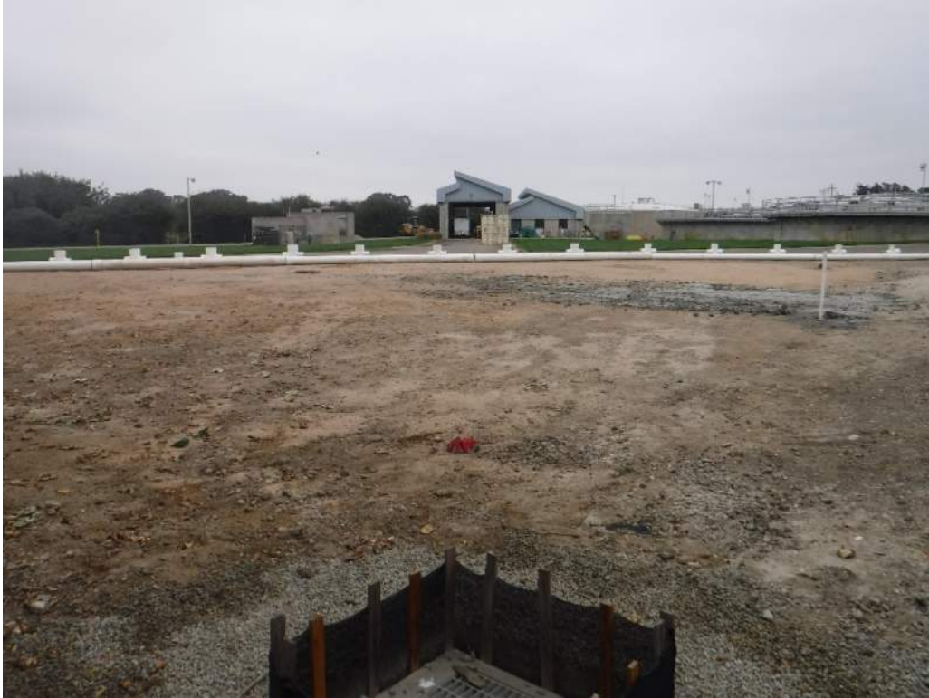
Photo 1 - East toward new Secondary Clarifier
