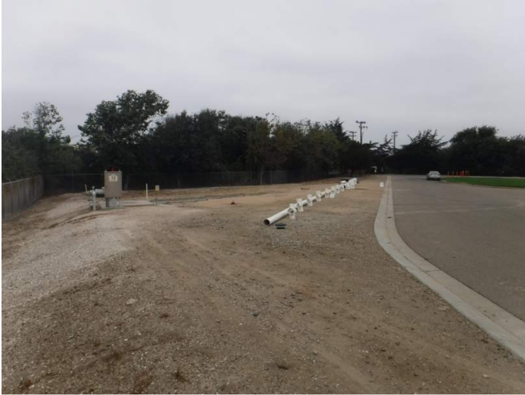
Photo 13 - North toward new Secondary Clarifier
