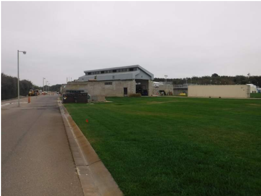
Photo 8 - South (slight east) toward existing utility (new Aeration Basin on far right of photo)
