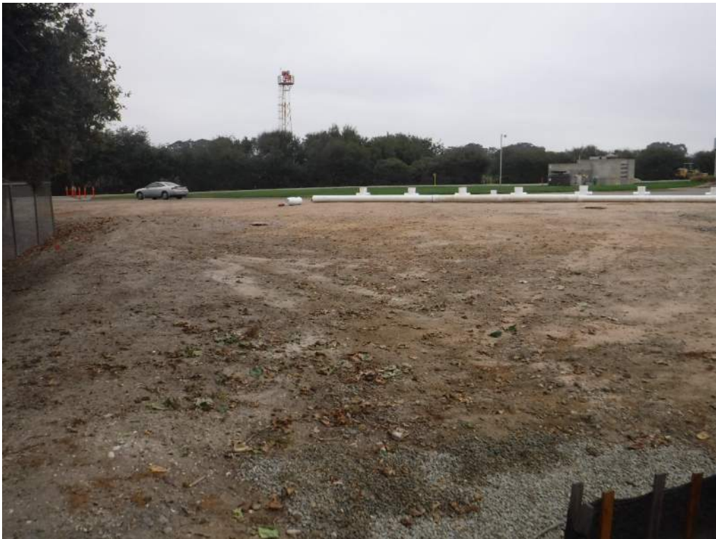
Photo 2 - East (slight north) toward new Secondary Clarifier
