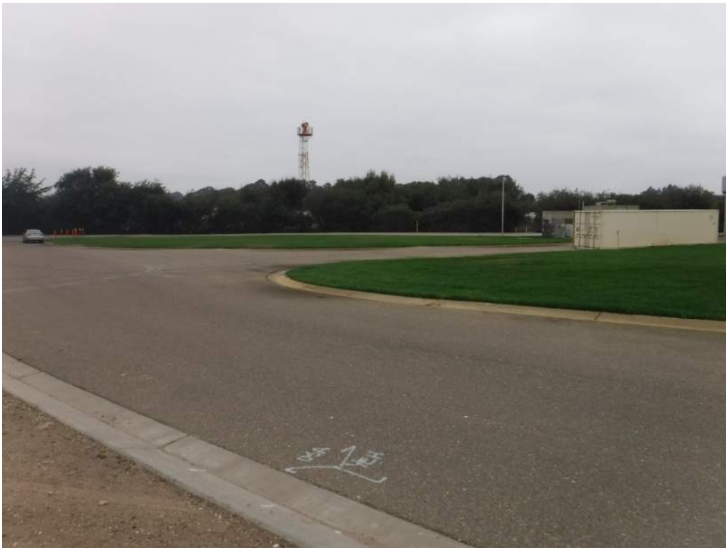
Photo 14 - North (slight east) toward new Secondary Clarifier and new Aeration Basin
