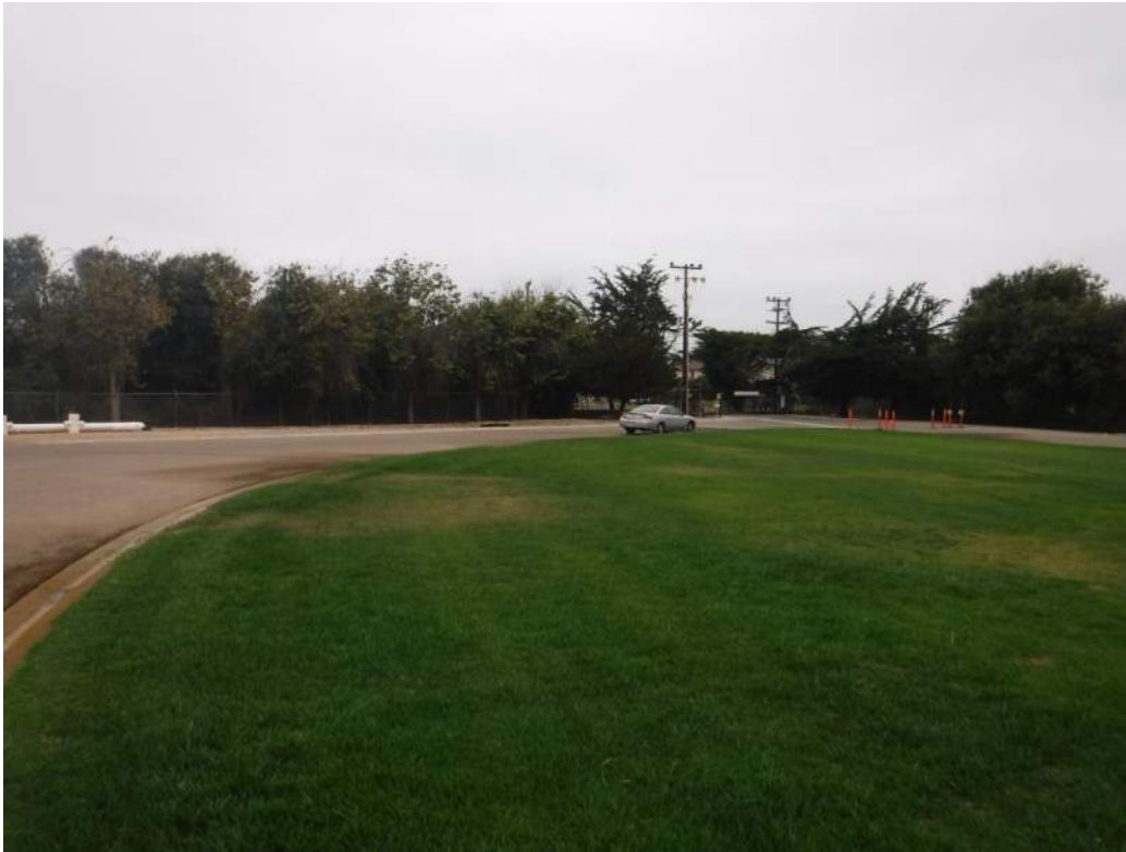
Photo 6 - West (slight north) toward new Secondary Clarifier
