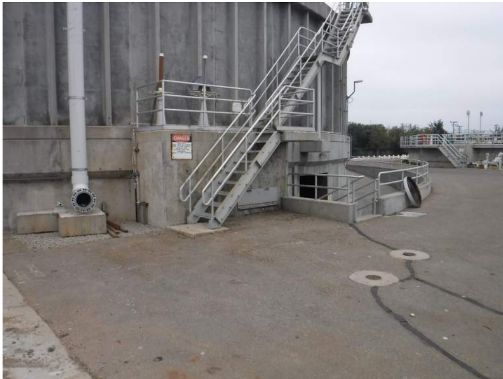
Photo 16 - North (west) toward new Fixed Film Reactor Effluent Pump Station
