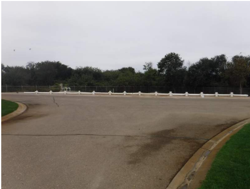
Photo 4 - West toward new Secondary Clarifier
