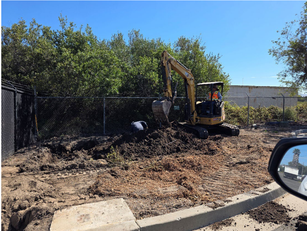
Operators Justin Musick and Mario De Leon excavating to remove old sprinkler water line.
