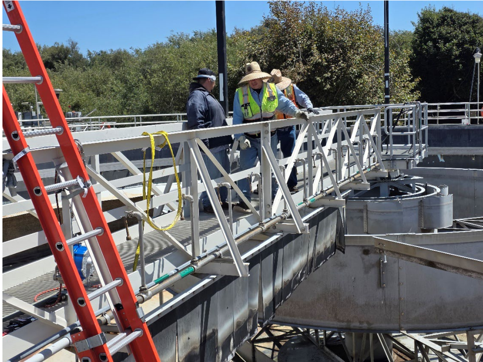
Operators Mario De Leon, Everardo Vargas, and Justin Musick preparing Secondary Clarifier No. 1 for operation.
