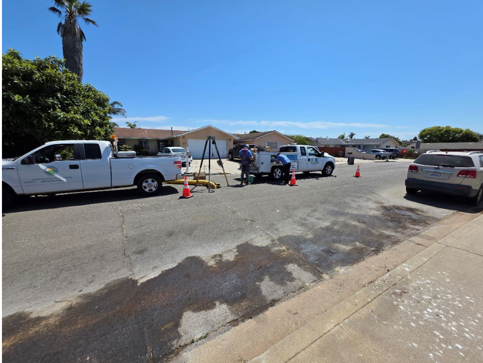
Gold Coast Environmental performing a confined space entry to install new permanent flow/velocity meters in District trunk sewer system.
