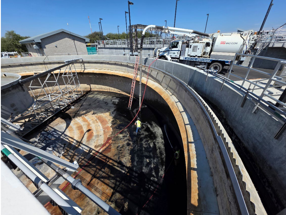
Fluid Resource Management performing the cleanout of Secondary Clarifier No. 2.
