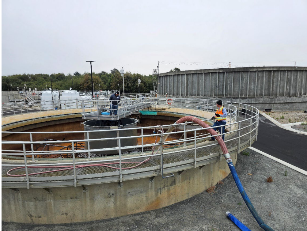
Justin Music and Mario De Leon observing the pump out of Secondary Clarifier No. 2 into Primary Clarifier No. 2.
