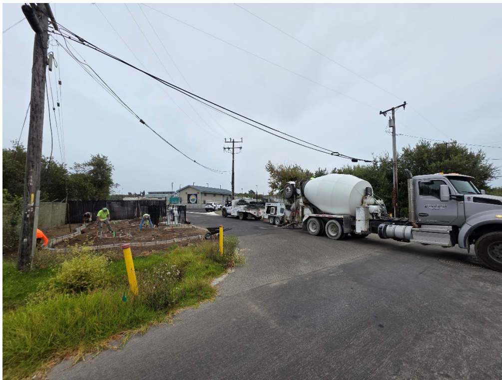
JNE Concrete pouring concrete landscape curbing
