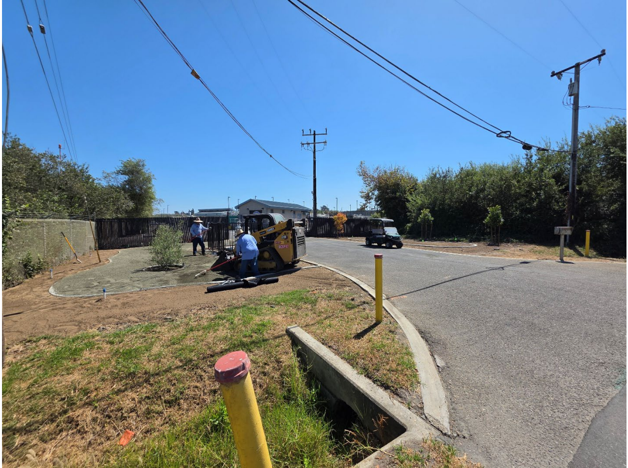
Operators Mario De Leon and Justin Musick continue their work on the front entry landscaping project.
