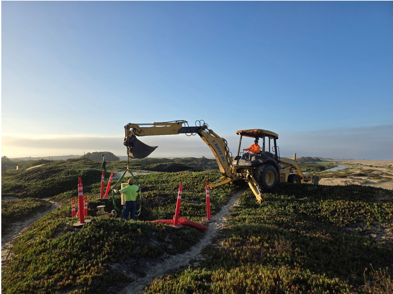
R. Baker Inc. performing the removal of the District's outfall junction box hatch.
